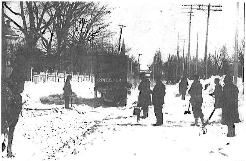
BELOW: A snow sweeper at work on Cote des Neiges, just north of Sherbrooke street, about 1900. This is one of ten sweepers built by the MSR in its own shops in 1898 and 1899. Snow shovels are much in evidence since in spite of the mechanization there was still a great deal of hand work required to keep the lines open after a big snow storm.
