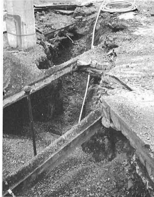
Relics of the past. Street car rails uncovered on Cote des Neiges road on June 13, 2000. In the background of the left photo behind the church (demolished in 2001) is the location of the original street car line used from 1899 to 1917. Photos by Fred Angus
