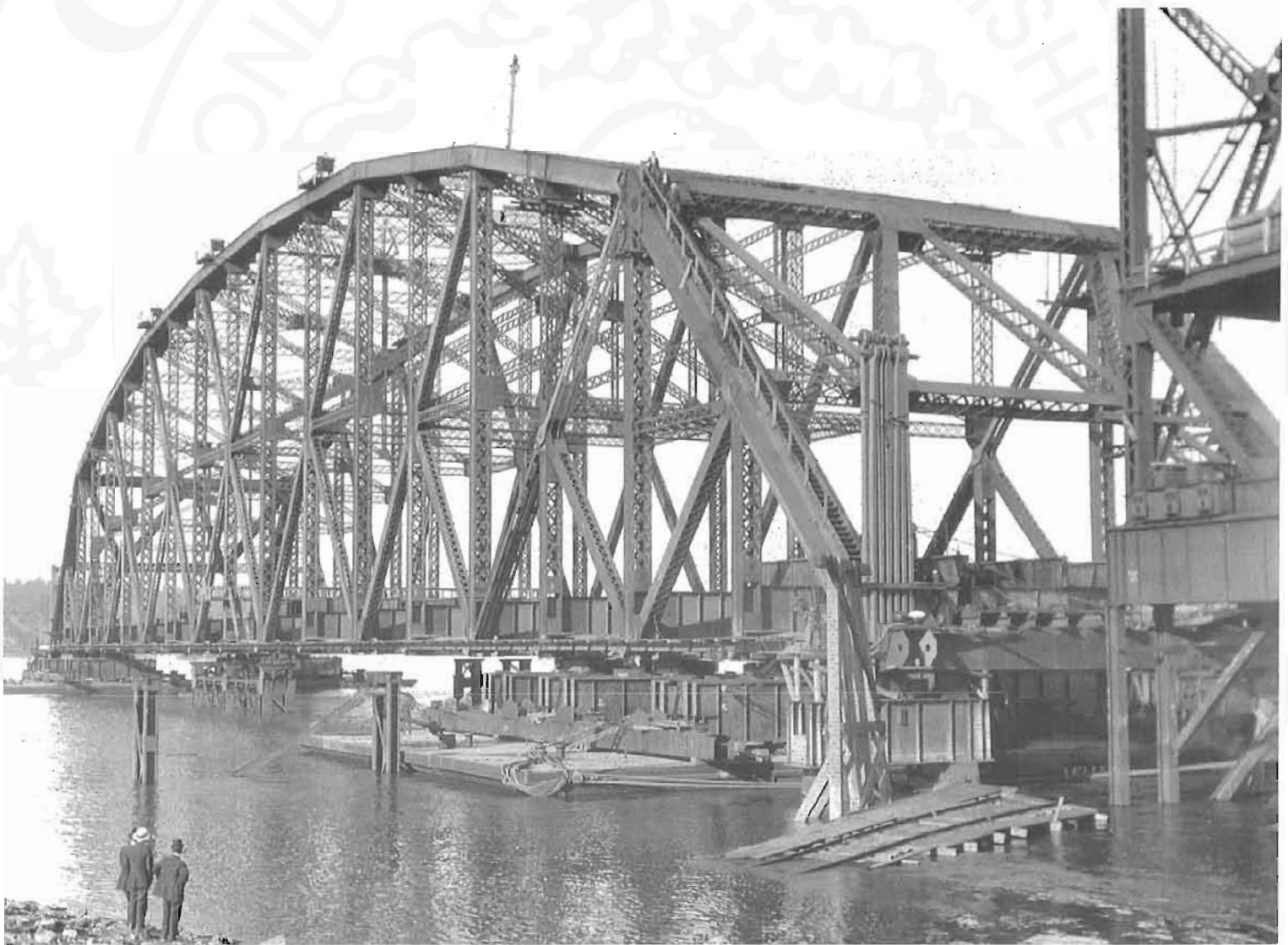
QUEBEC BRIDGE CENTRE SPAN SEPTEMBER 10 1916
