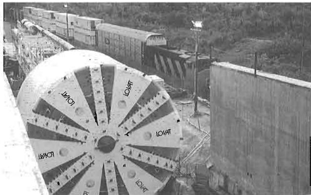
"Excalibore" about to start drilling the new St. Clair tunnel, September 16, 1993.
