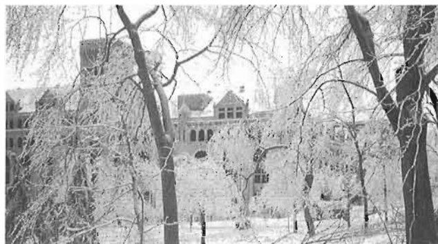
Windsor station during the ice storm. January 9, 1998.
