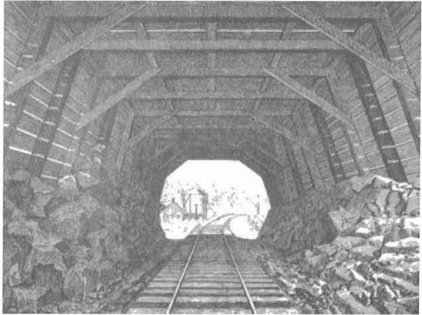
Another snowshed on the Intercolonial was this one near Campbellton. Courtesy of New Brunswick Museum
