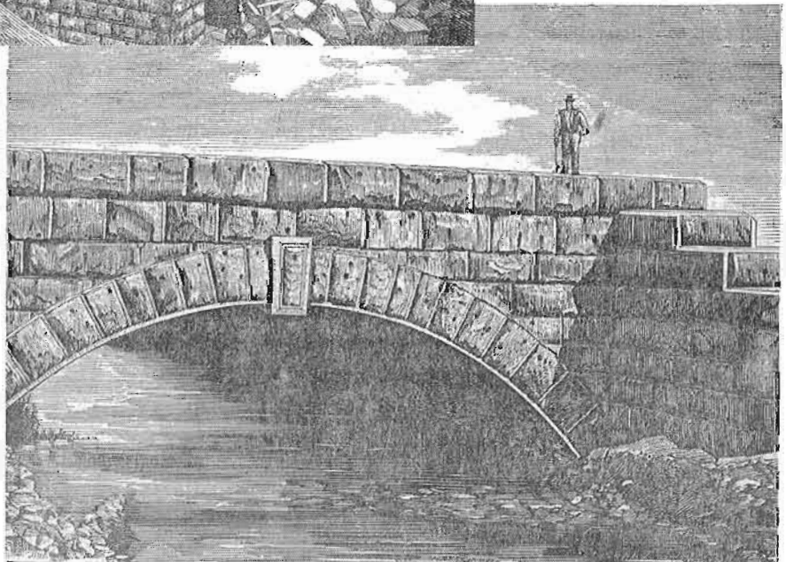
RIGHT: The cut stone culvert over the Kouchibouguac river in 1874, before the railway embankment was built on top of it.
