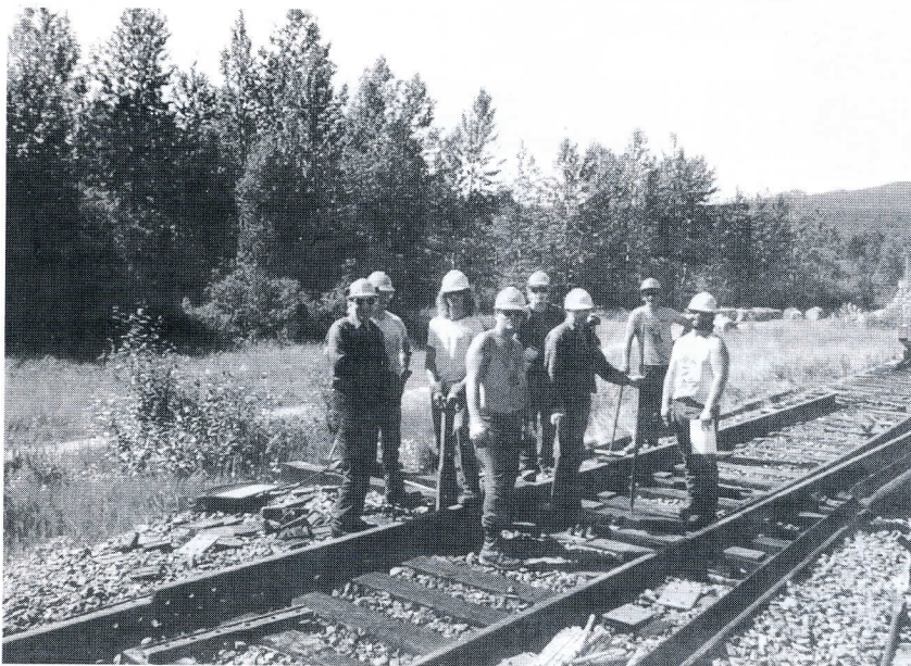
Photographers of railway subjects seemed to have ignored section gangs at work as a topic, author included, and this is the only one he has been able to locate. Here two gangs, from McBride, [Mile 0.0] and Dome Creek [Mile 55.7], work together to replace a switch connection at Goat River [Mile 27.8] on the CNR Northern BC Line, in 1988. Prince George is another 118 rail miles to the west. Hard hats had become mandatory headwear. Jim Harte
