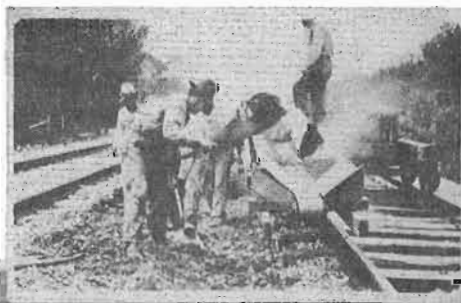
The HARRIS-MUFF Ballast Screening Machine in Operation.
