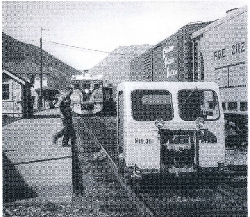
Lillooet station in 1964 on the Pacific Great Eastern Railway [now BC Rail], being the upper terminal of a daily passenger service from North Vancouver. The Budd car train is about to return southwards and is being preceded by a speeder for the next 35 miles because of constant threats of rockfalls.
