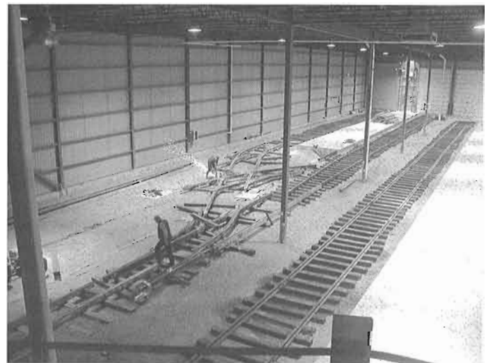
ABOVE, ABOVE RIGHT AND RIGHT: Three views of volunteers laying track in the new building. The tramways track is from the former St. Henri carbarn.
