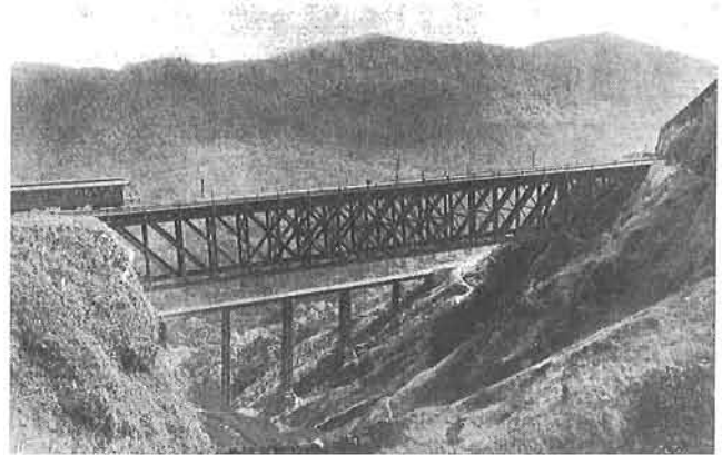
The Mogy viaducts on the Sao Paulo Railway of Brazil. Light engineered these spans with his student Henry Ketchum.
