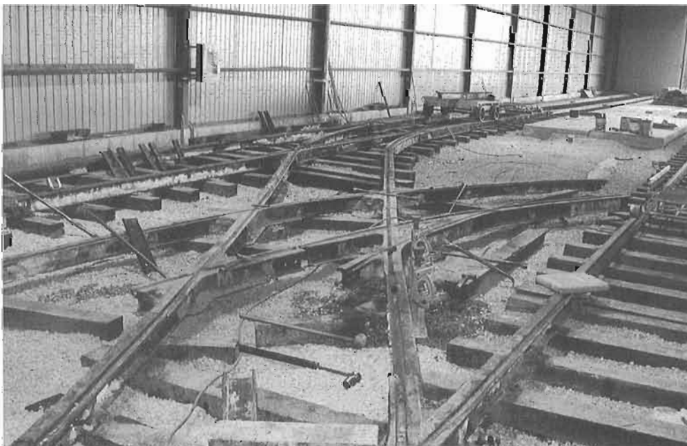
LEFT / GAUCHE: Overall view of street car special work. (PM)
