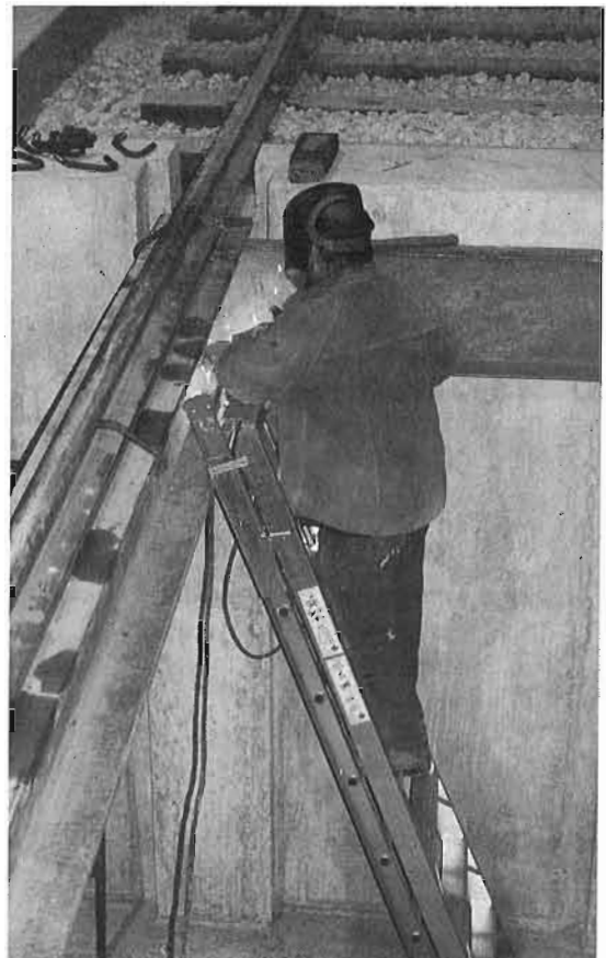
Welder installing steel cross bracing between the rail support beams. (PM)
