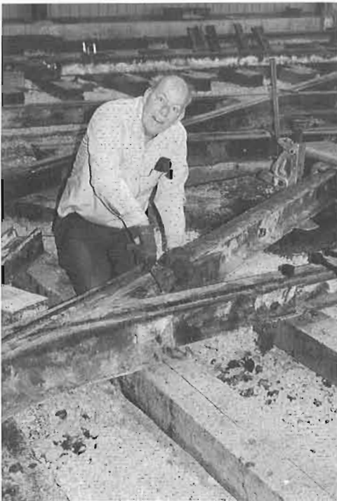
Gord Hill, (volunteer and retired STM employee) instigator of the streetcar special work making a final tie in. (PM)
