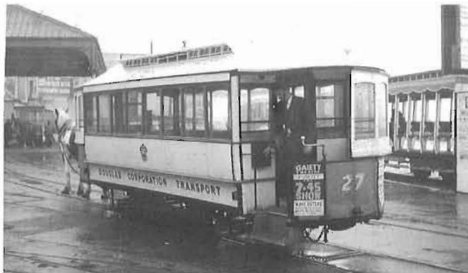
Two views of Douglas Corporation Transport car 27. This car, along with Nos. 28 and 29, were built by G.F. Milnes of Birkenhead England in 1892. These three cars are virtually as built and the most authentic examples of horsecar construction in service anywhere. They are usually used in rainy weather when the open cars remain in the barn. All IOM photos by Fred Angus.
