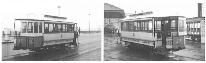
Two views of Douglas Corporation Transport car 27. This car, along with Nos. 28 and 29, were built by G.F. Milnes of Birkenhead England in 1892. These three cars are virtually as built and the most authentic examples of horsecar construction in servive anywhere. They are usually used in rainy weather when the open cars remain in the barn. All IOM photos by Fred Angus.
