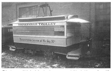
This strange vehicle is obviously a horsecar converted to electric operation, while still retaining its pedestals. Amazingly it was photographed as recently as November 21 1943 in Kitchener Ontario. It was probably a passenger car of the Berlin & Waterloo Street Railway, later used as a work car. Its final disposition is unknown. National Archives of Canada, Merrilees Collection, photo No. PA-166504.
