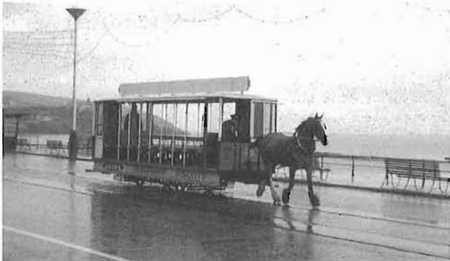
Car No. 49 is one of three convertible cars built in 1935, the newest cars in the Douglas horsecar fleet. They are open cars which can be converted to closed in bad weather.
