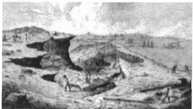
Cutting the roadbed for the Western Extension's Carleton branch which ran down to the west side of Saint John harbour. The downtown core of the city on the opposite side of the harbour is visible in the background. During its lifetime (1869-83) the CIN published many illustrations of early Canadian railways, all of which may be found in the National Library's online database of CIN images at <www.nlc-bnc.ca/cin>
