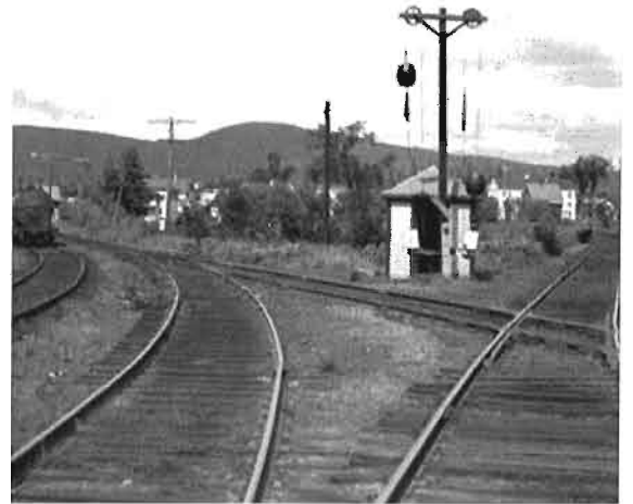
An old fashioned ball signal explains the origin of the term "highball".
