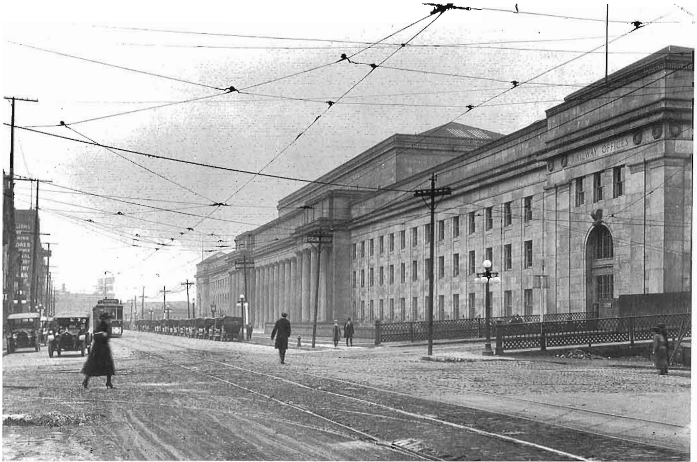
Toronto Union Station finally opened in 1927 after years of delay. This photo was taken during the 1920s. Canadian Pacific Corporate Archives, photo No. 11305
