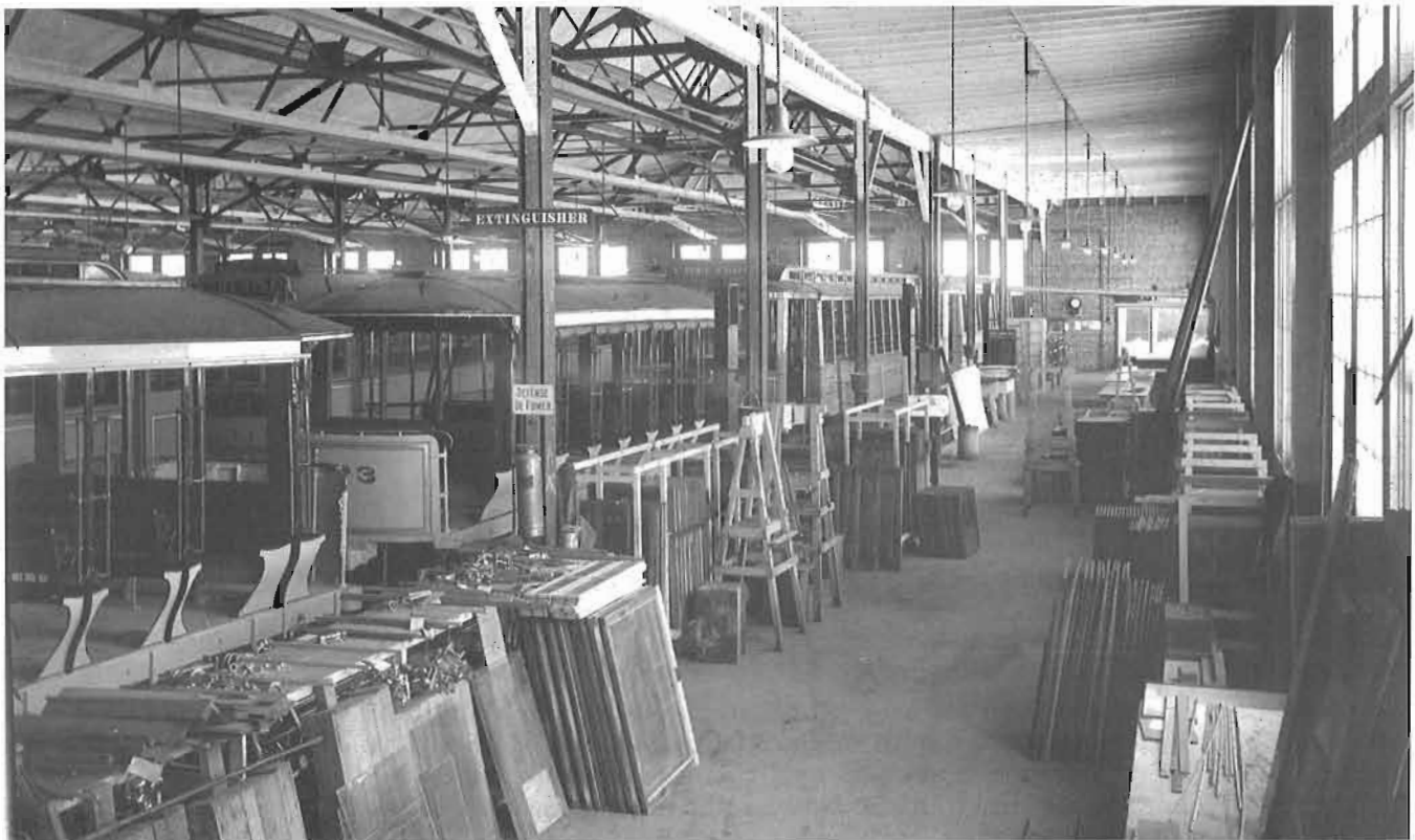
Some 651 class cars awaiting conversion to closed cars in 1912. Also two large 703 class Pay As You Enter cars awaiting repairs. Note the blackboard with the car numbers written thereon.
