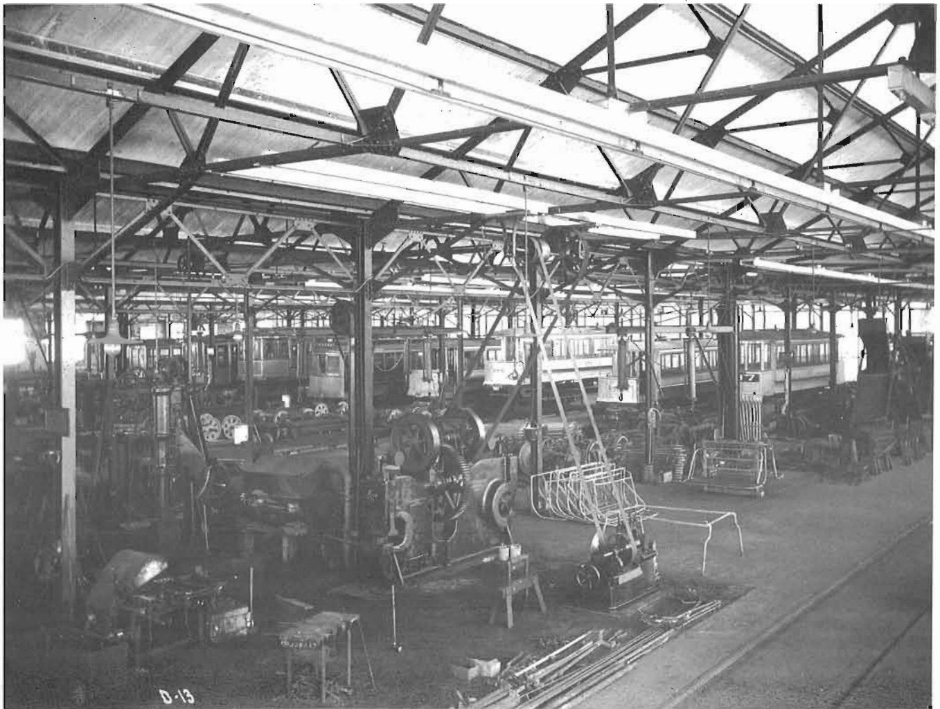
Interior view of main building, showing Blacksmith Shop, and overhauling space in the background. The 651 class open cars, built in 1901, are in the shops being converted to closed cars.
