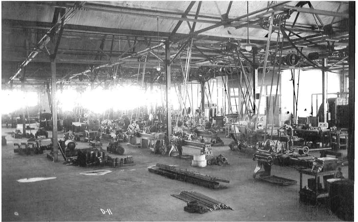
View of some of the lathes in the machine shop.
