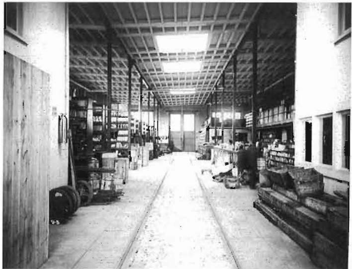
A view inside the Stores Department, showing the track from which it is supplied.
