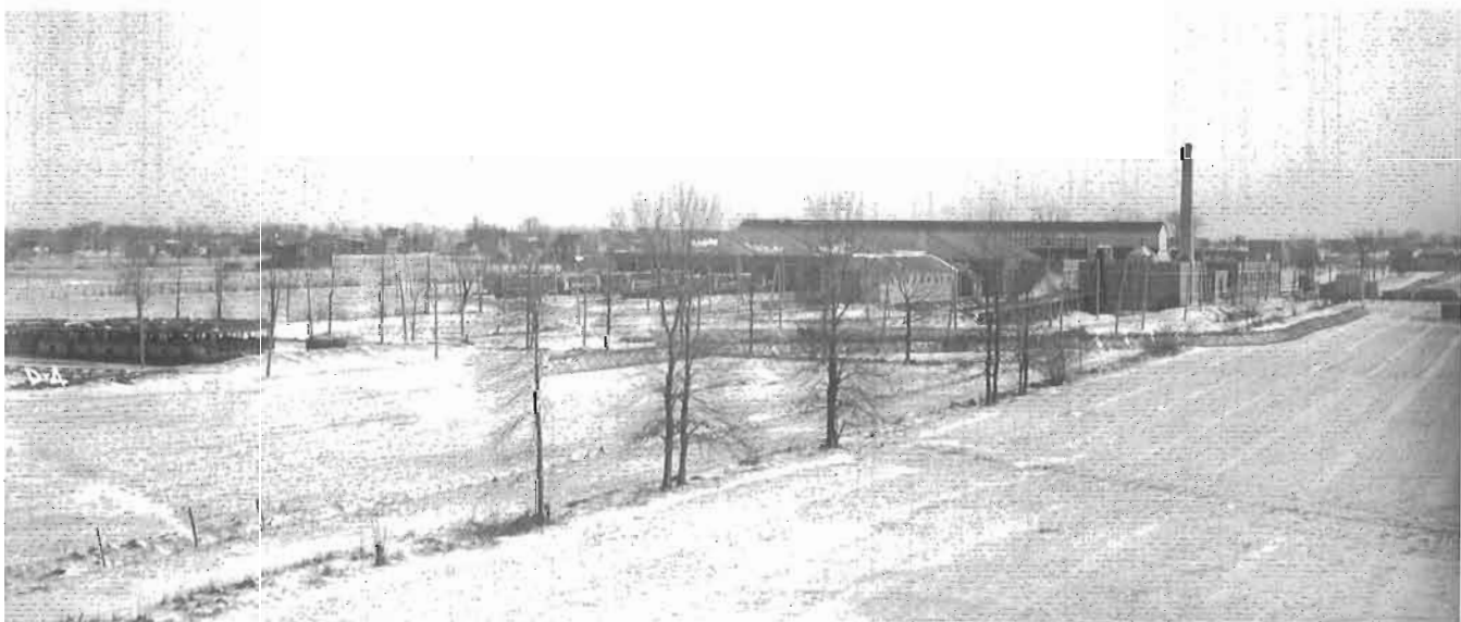
Three exterior photos of Youville Shops as photographed new in 1912. Note the old cars, of 1890s vintage, some of Montreal's earliest electric cars, outside the shops in the two top views. These cars were retired from passenger service about this time; most were scrapped but some were converted to work cars. On the left side of the bottom view can be seen the bodies of about a dozen open cars, built between 1893 and 1895. These were undoubtedly awaiting scrapping.
