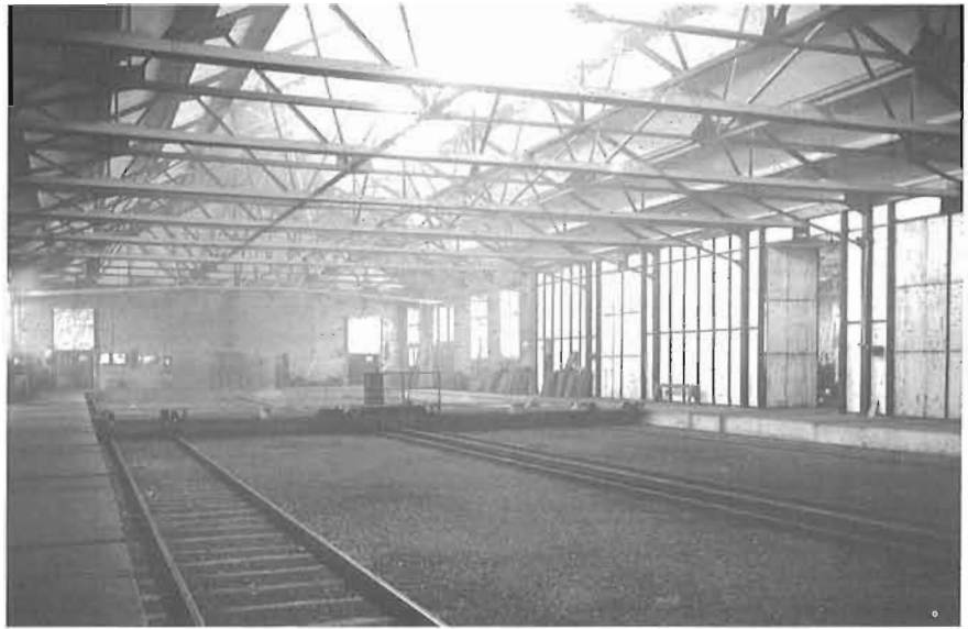
Covered-in transfer table which centrally divides the shops.
