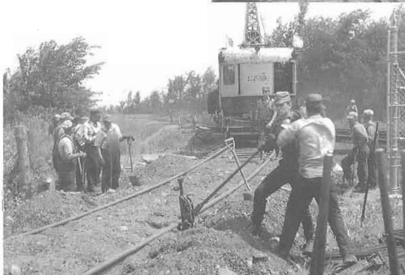
ABOVE AND LEFT: Twelve days later the trackwork was well advanced, and the CPR crew was hard at work, as can be seen from these views taken on July 10, 1962. Notice that the building is now completely sheathed. A few years later it was doubled in size.
