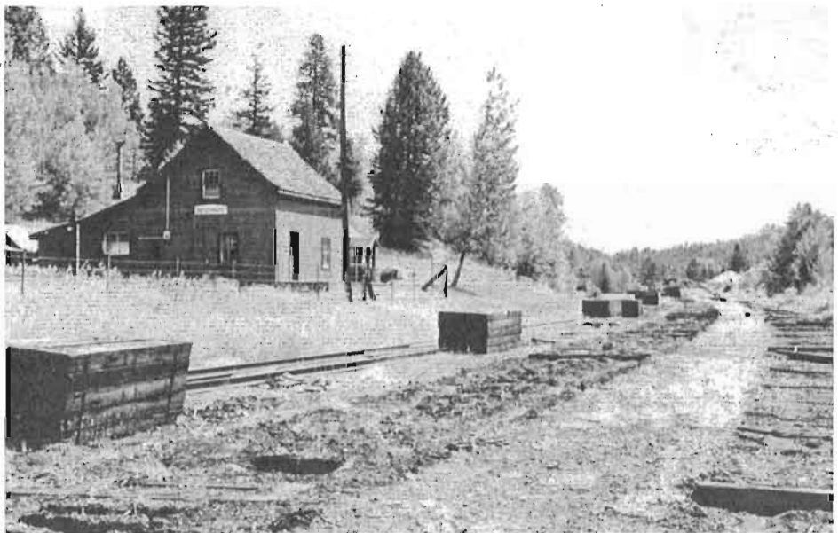
A good example of ties in differing conditions of quality. The bundled ties will be used by CPR somewhere else in western Canada, whilst those left in the grade will soon be removed and trashed. In the background is a former section house. Brookmere, August 1991.
