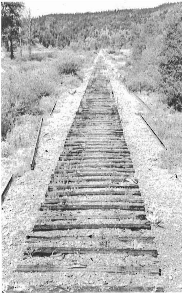
One hour earlier this was solid railway track capable of bearing a train. Now it is just a view of old ties in serried ranks.
