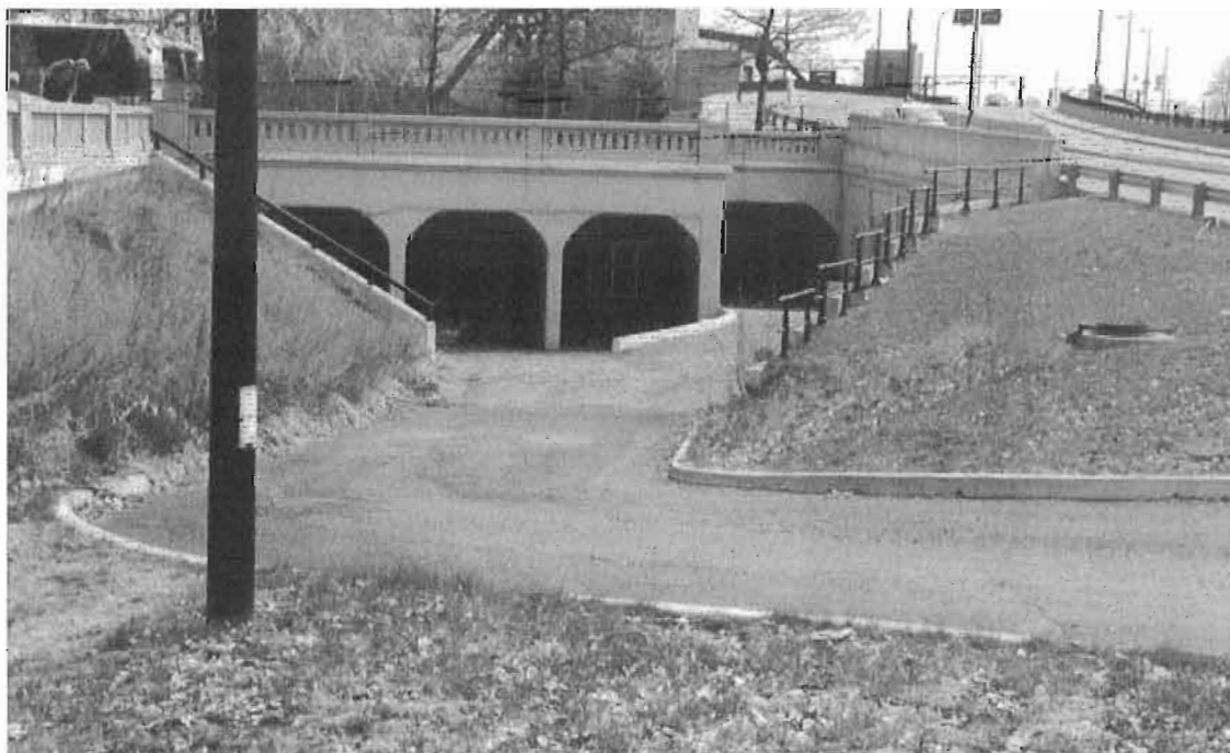
One of the tunnel portals as it appears today (2005). Photo by Peter Murphy
