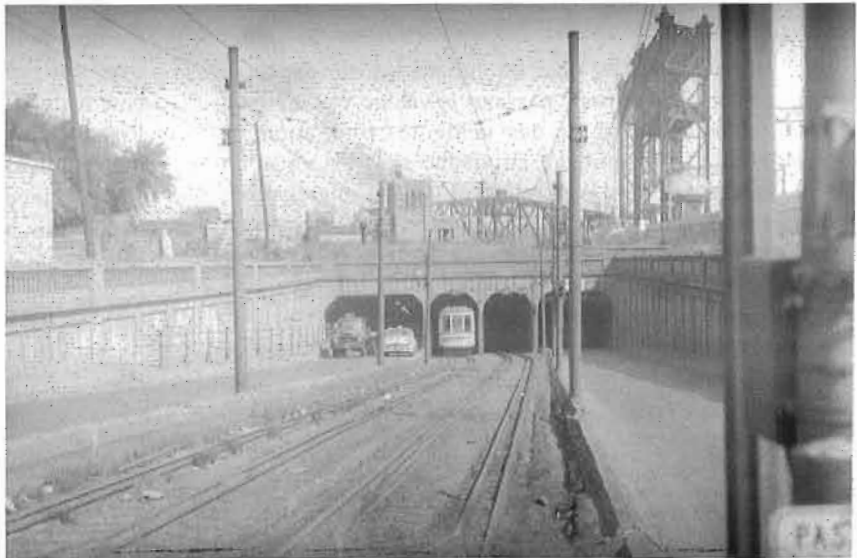
A 1600-class car emerging from the Wellington tunnel.
