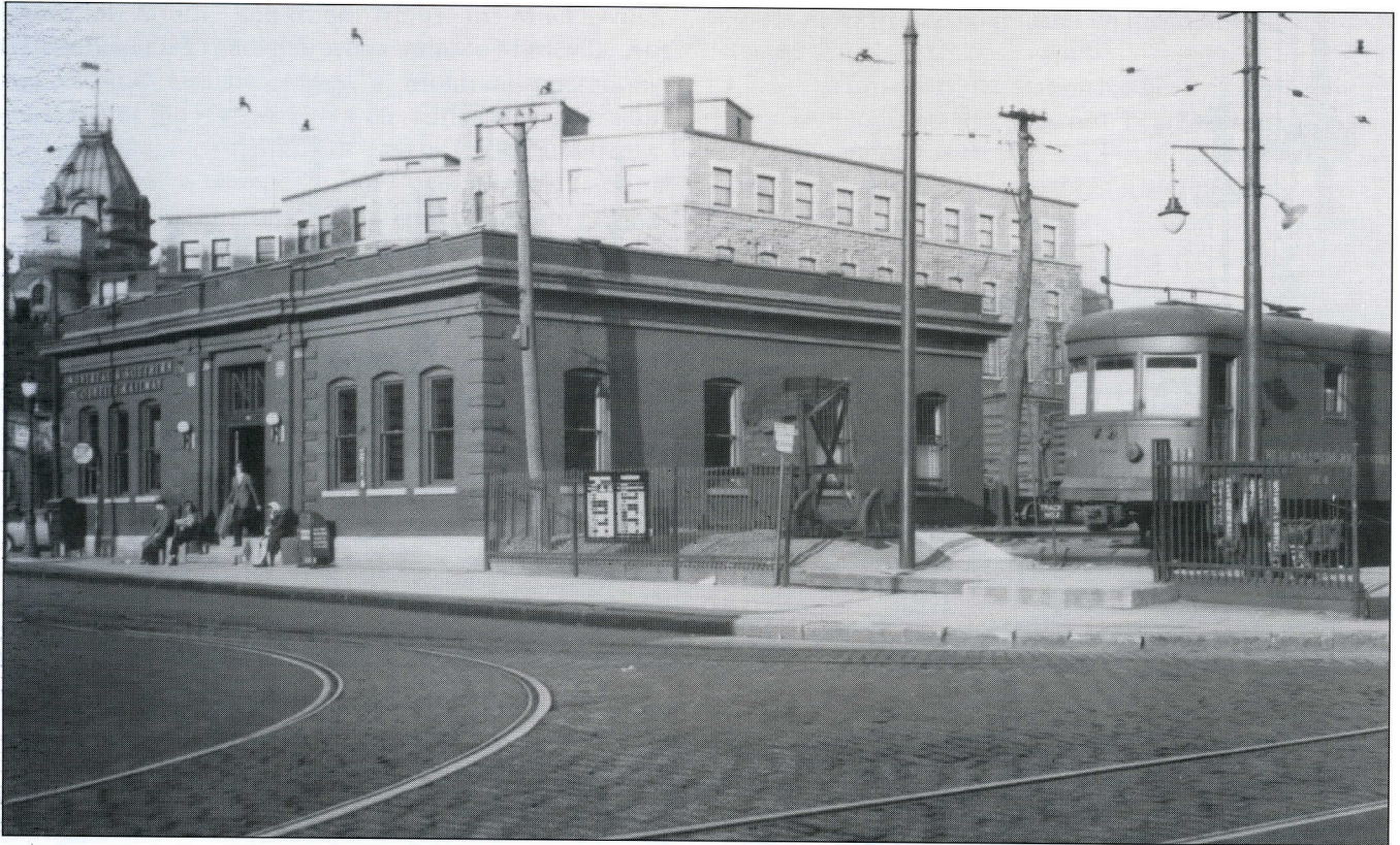
The McGill St. station on May 3, 1948. Note the old wye tracks in the foreground. Photo CRHA Archives, Fonds Corley.
