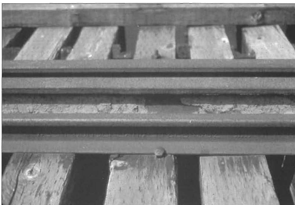
Thousands Islands Railway Guard Rail, West Cumberland Steel, 1882. Gananoque, Ontario, Canada, 22 June 1985. Photo #16338: Hugues W. Bonin.
