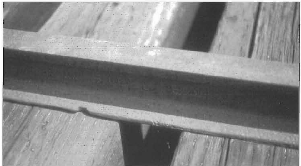
Thousands Islands Railway Guard Rail, Barrow Steel 74 lbs, 1872. Gananoque, Ontario, Canada, 22 June 1985. Photo #16346: Hugues W. Bonin.
