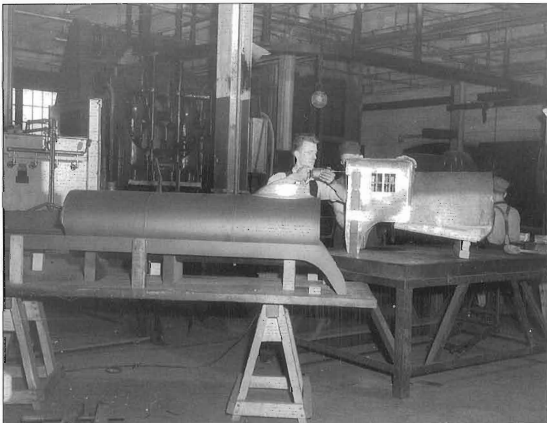
Workers building the boiler and cab assembly at Angus shops. Photo CPR Archives.
