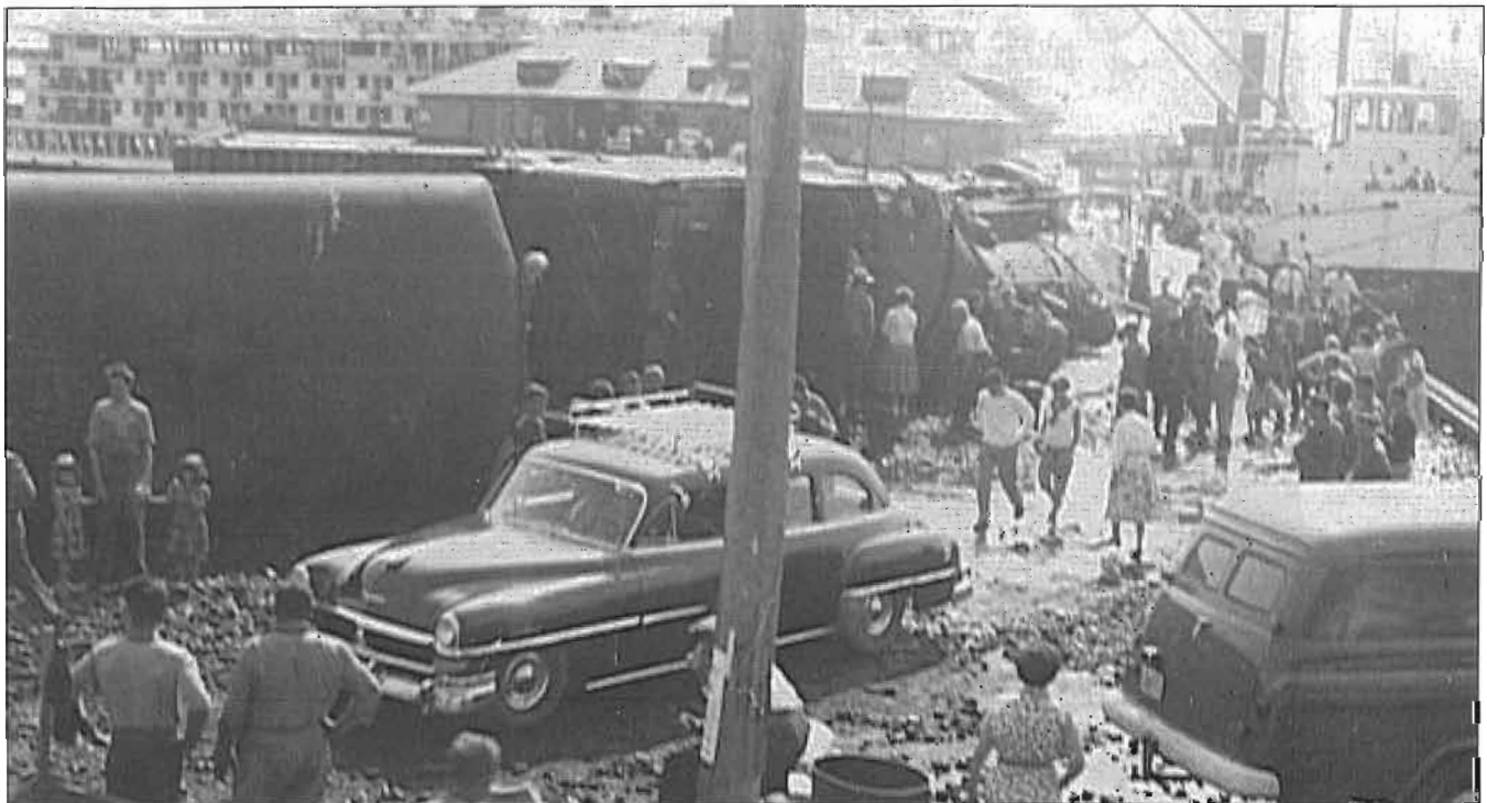
The derail frog in fact derailed the locomotive preventing it from hitting the white ship Richelieu from the Canadian Steamship Lines, with 100 passengers on board.
