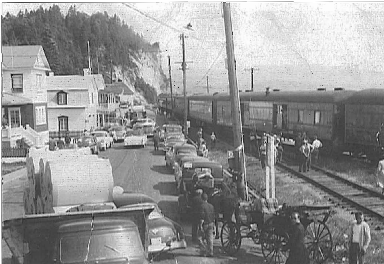
The switch not being replaced in the proper position by the section man.
