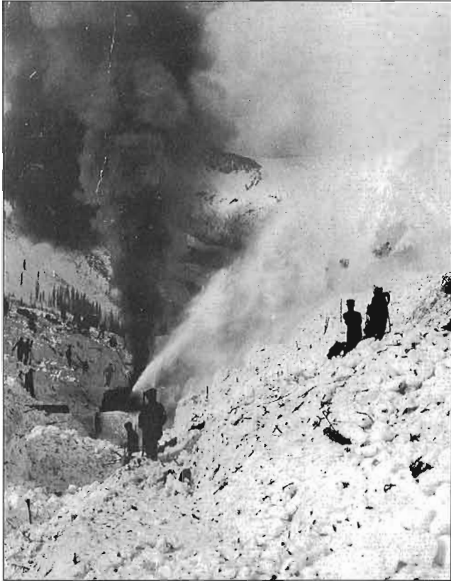
A rotary attempting to clear the line after a snowslide in 1910. Debris mixed with the snow could cause damage to the plough's blades and other equipment. Photo, Canadian Pacific
