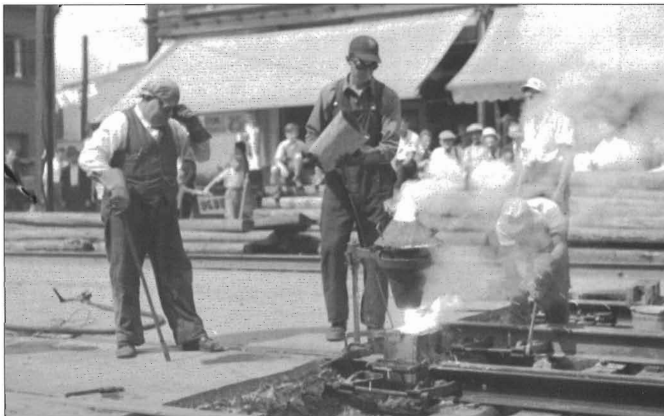
MTC Employees welding rails on Notre-Dame Street in Montreal, August 1939
