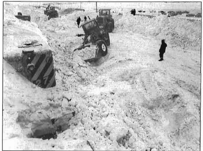
In the diesel era snow still blocks the lines and buries trains. However, bulldozers and front loaders are now frequently used to remove snow, as we see in this scene taken in 1979. As a result, the use of the traditional snow plough is diminishing. Photo, Canadian Pacific
