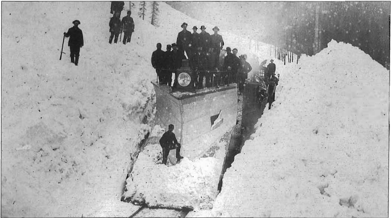
The equipment was a bit different but the conditions much the same in the early days. Here we see a wooden CPR plough paused for a photograph in the mountains, probably in the 1890s. Note the oil headlight in a rather vulnerable position atop the plough. Photo, Canadian Pacific
