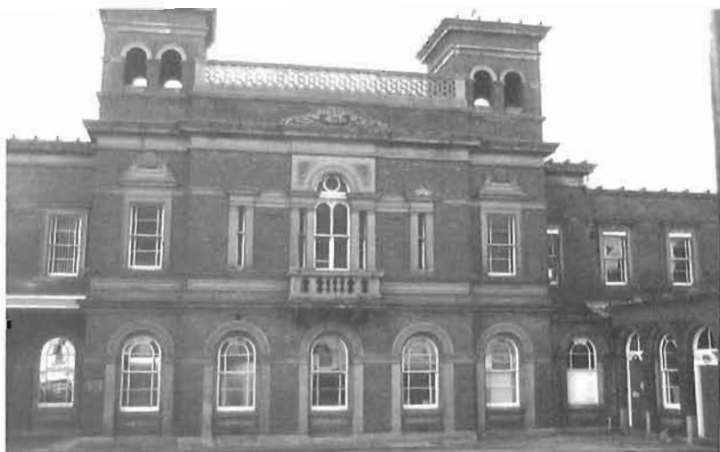
Chester station, on the Chester & Holyhead Railway, was also designed by Thompson. The multiple arches are also very prominent in this structure. This is the oldest surviving Italianate-style station in Britain. David Jeanes
