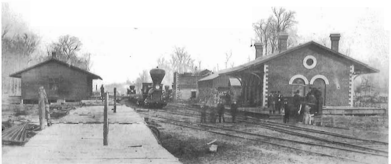
A lively scene at Mount Clemens Michigan about 1860. The station is a brick type "C" structure with five bays. This station is still standing. National Archives of Canada, photo PA-138693.
