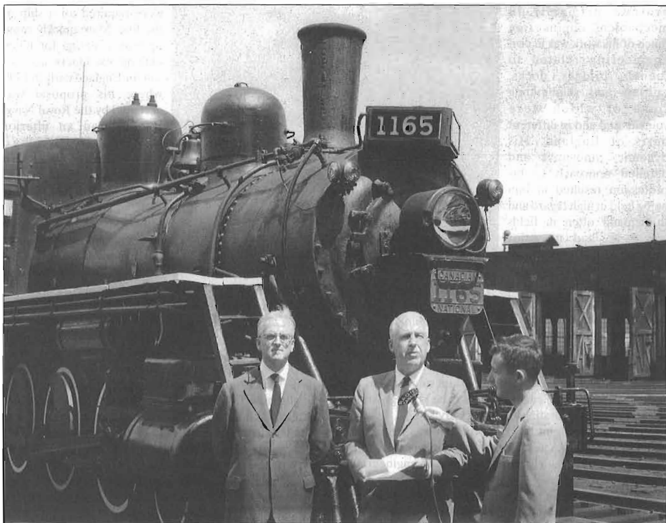
Dr. Robert Nicholls accepts the donation of CNR 4-6-0 steam locomotive 1165 in 1960 on behalf of the CRHA. This was the first CNR locomotive preserved by the Association, it was re-numbered to 1009 (its original number) and is on loan to the Salem & Hillsborough Railway (New Brunswick Division of the CRHA). Photo CRHA Archives courtesy Josee Vallerand archivist.
