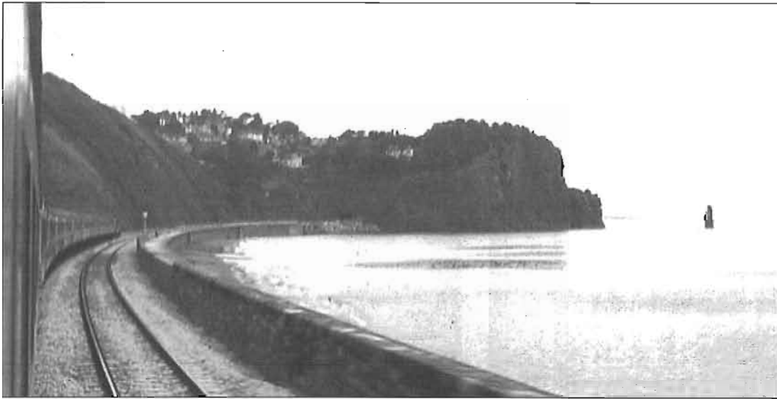
A view of the former Great Western line along the Devon coast. Near here was the site of Brunel's most spectacular failure, the Atmospheric Railway of 1848. Photo by Fred Angus
