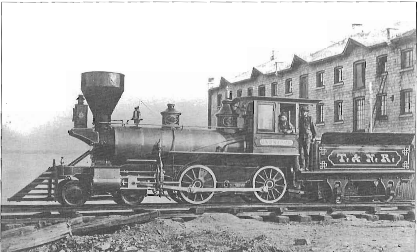
Official photo of the Toronto & Nipissing's No. 6 'Uxbridge' taken at the Canadian Engine and Machine Company works in Kingston, Ontario in 1871. Note the light narrow gauge track laid upon inverted 'U' rail broad gauge siding. Photo CPR Archives No. A112, CRHA Archives, Fond Corley. Copyright © 2005
