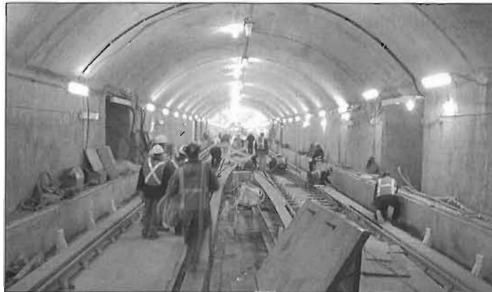
Installation of a double cross-over in the new tunnel to Laval.
