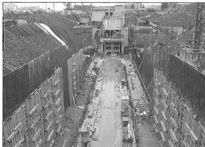
The Cartier station under construction in 2005.
