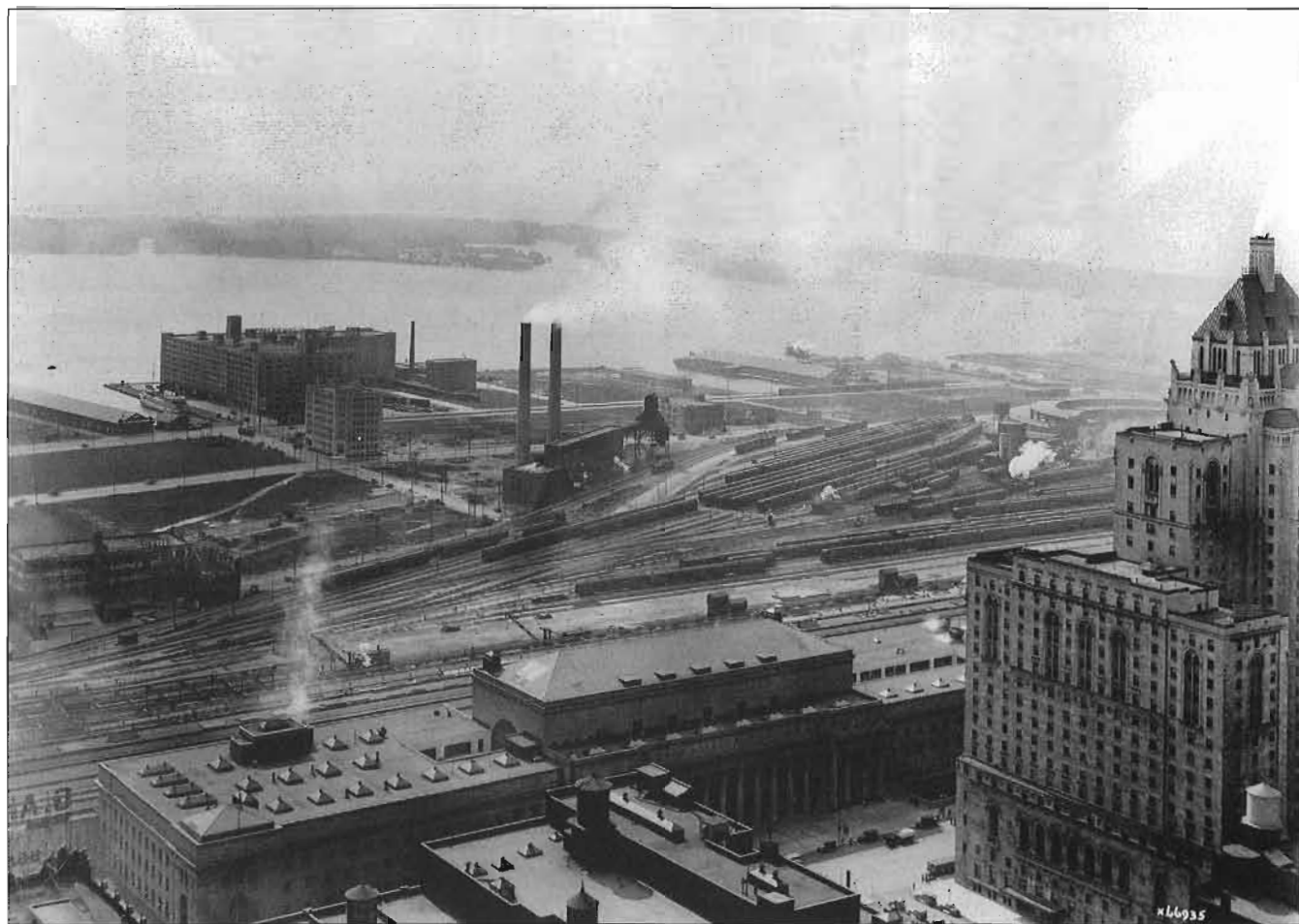
The two chimneys left of centre delineate the Toronto Terminals Railway Central Heating Plant in this 1930 view. On the right are the Canadian Pacific Railway's John Street roundhouse and Royal York Hotel, both opened in 1929. Archives of Ontario 10002016
