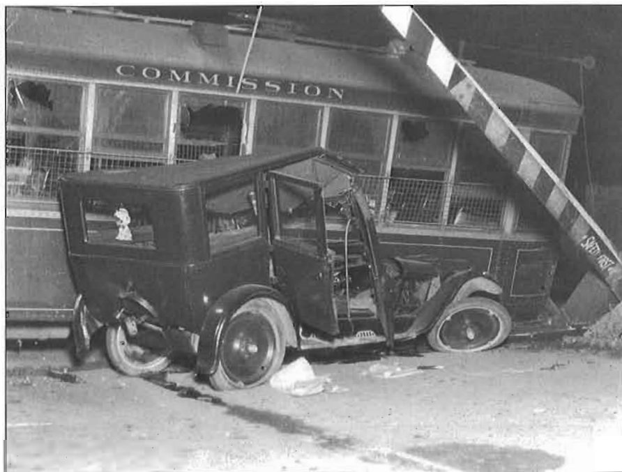
The necessity for the railway viaduct was underscored by this 1926 accident at the Queen Street level crossing. Runaway CN freight cars collided with a TTC Peter Witt streetcar, which then slammed into this automobile. City of Toronto Archives, Fonds 1266, Item 8780
