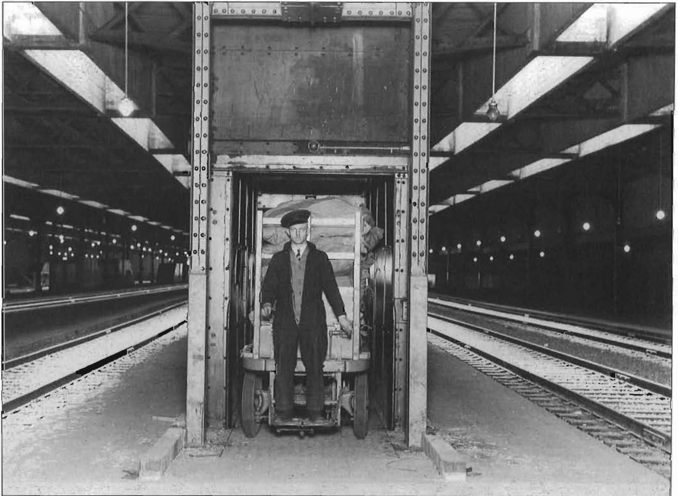
These battery powered baggage wagons were built in 1929 to transfer baggage between the basement and the platforms. Amazingly, some of them are still in use in 2007. City of Toronto Archives, SC 367, Item 16
