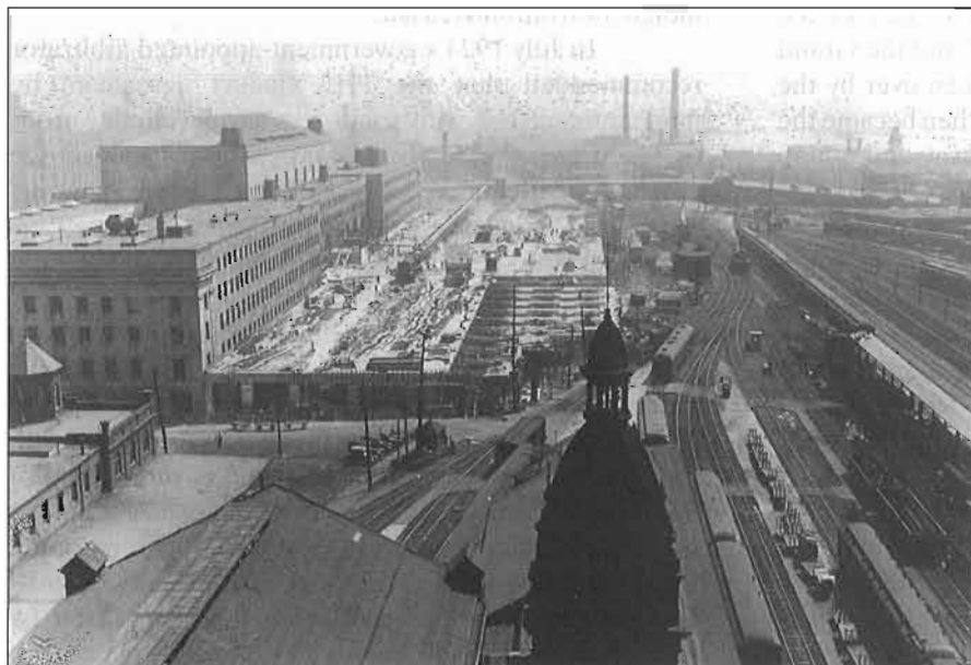
The most complicated aspect of the grade separation project was the viaduct structure located between York Street and Bay Street. This early 1927 view was taken from the centre clock tower of the old Union Station. City of Toronto Archives, Series 372, Sub-Series 79, Item 244
