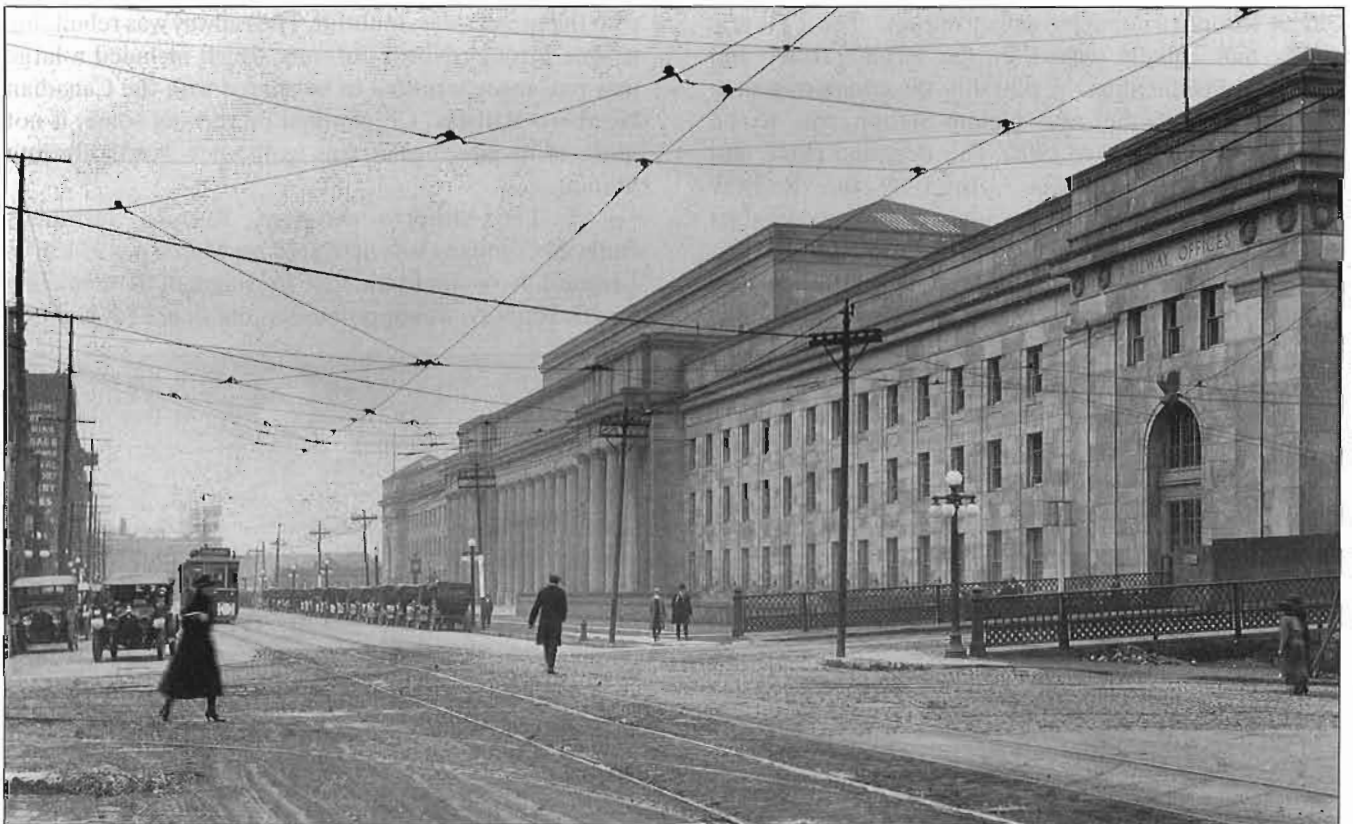
This view of Toronto Union Station is looking east along Front Street in the early 1920s. The headhouse has been completed and the railways have occupied the offices in the west wing. The centre block containing the actual passenger station facilities sits empty while various levels of government and the railways argue about how to build the tracks into the station. Photo Collection Frederick Angus.
