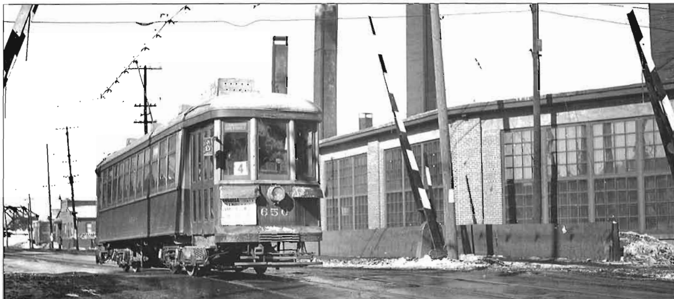
Car #650, one of six cars (650-655) built by the QRL&P in 1916, can be seen crossing the CPR tracks and passing the CPR roundhouse on de la Couronne St. in March 1946. This car was originally built as a two-man pay-as-you-enter (PAYE) car but was later converted by the company to a one-man car. Note the manual level crossing and the reinforced trolley wire over the CPR tracks. Ernest Modler, Ronald S. Ritchie Collection.
