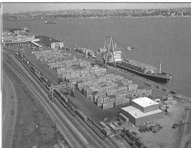
Aerial view of the container terminal at Wolfe's Cove as it appeared on April 26, 1972. Canadian Pacific Archives E 2137-22.
