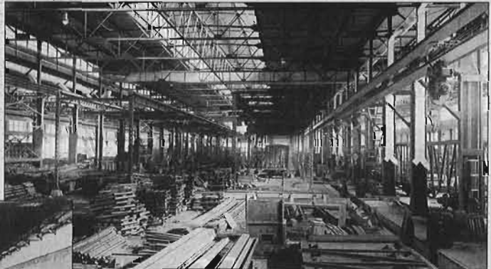
The erecting shop at the Eastern Car Company in 1916. CRHA archives.
