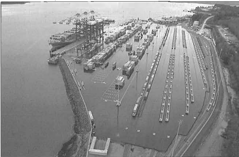
Further view of the terminal on November 1, 2007. First vessel Cosco Antwerp, 5500 TEU vessel owned by China Ocean Shipping Company, on the berth. CN Rail.
