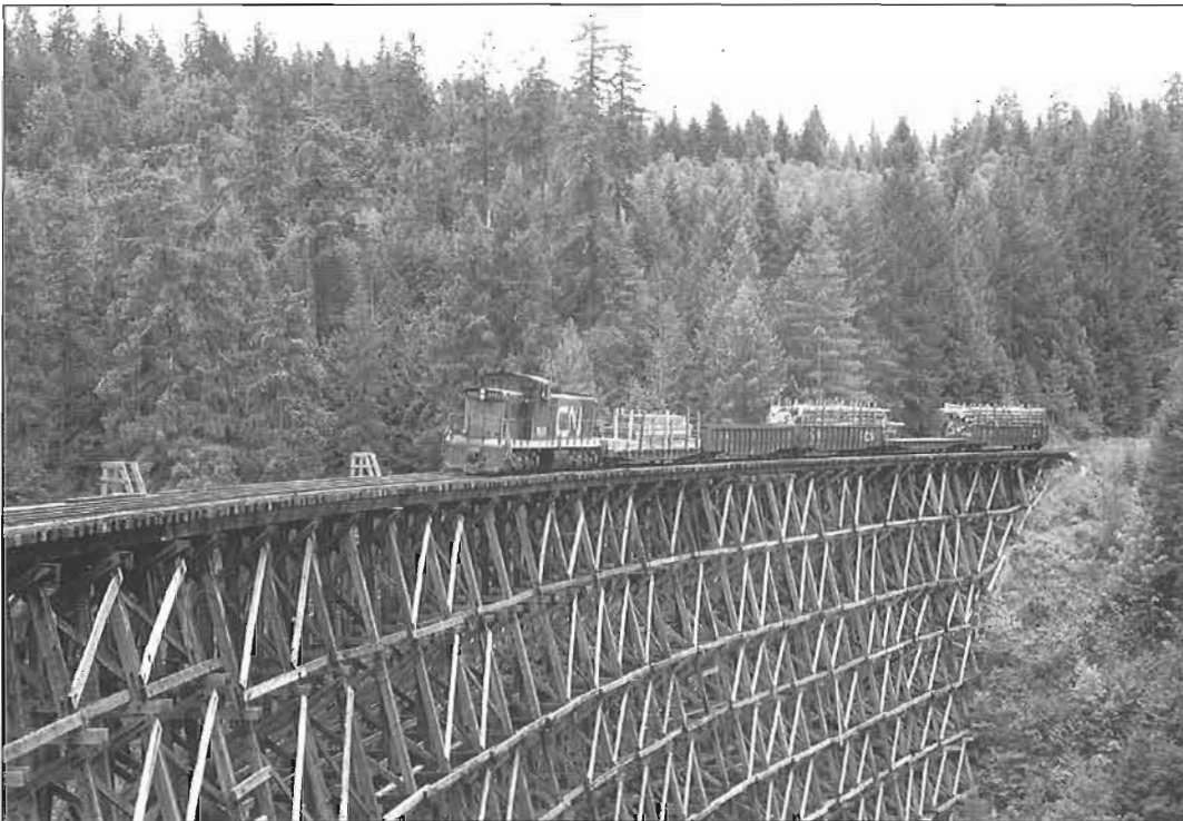
Canadian National No. 1000 and five cars was the last train over the Kinsol Trestle on June 20, 1979. The trestle was located at mile 51.1 on the Cowichan Subdivision on Vancouver Island. Dave Wilkie collection, West Coast Railway Association Archives.
