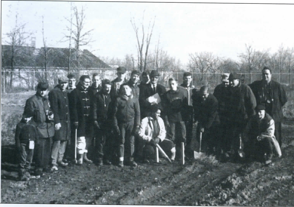
Group photo for the turning of the first sod for the construction of Building 2. We can identify the following: From right to left, Stephen Walbridge kneeling, Omer Lavallee behind him, the late Jack Beatty with his cigar, Donald Angus with the shovel, Dennis Peters to his left, Wyatt Webb holding stake in front, Robert Cox back row with engineers hat, Edward Plant and Walter Bedbrook second and third from left, Ron Bryant fifth from left. CRHA Archives.
