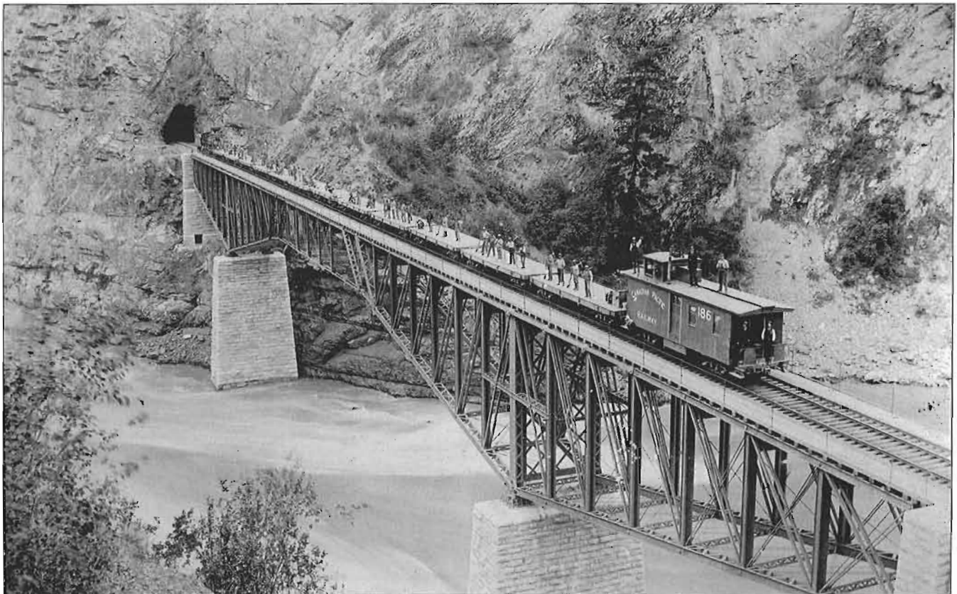
This photo appropriately titled 'Cantilever Bridge nr Cisco', the view is looking railway west (geographic south) with the tunnel portal in view. Canadian pacific railway has posed the train with what looks like the workmen and their tools, date unknown. CPR Archives # a11416
