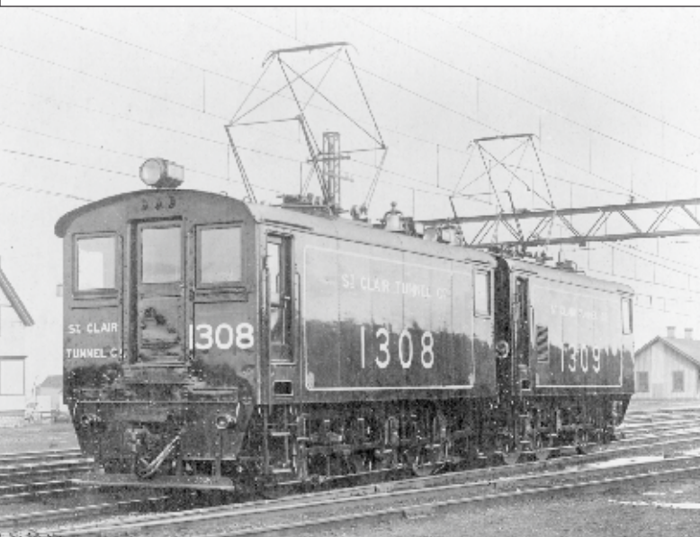
A pair of St. Clair Tunnel Company electric 'tunnel haulers' shortly after delivery in 1908. Electric Railway Journal enhanced by Paul McGee.
