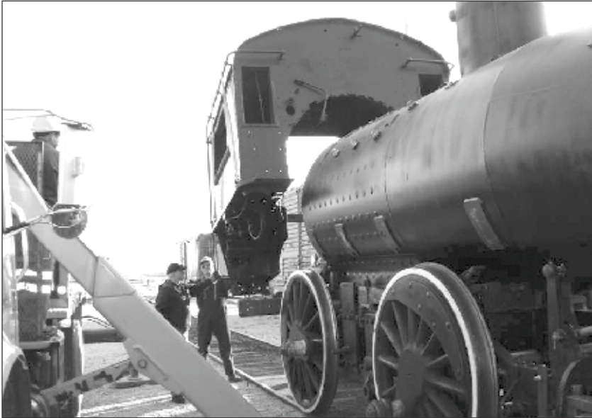
By early 2007 the cab had been reinstalled and the insulation and boiler lagging applied, old No. 3 was beginning to look like her old self! Paul Newsome.
