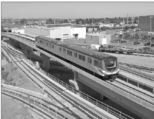
Cars 104-204 are southbound on the elevated guideway above the Operations & Maintenance Centre in Richmond on June 30, looking east from the Oak Street Bridge.
