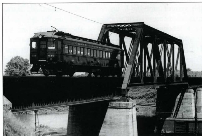
Grand River Railway 846 crosses the Waterford trestle in July 1947. The bridge was built in 1916 and crosses the Canada Southern Railway. M. D. McCarter N3806, CRHA Archives, Fonds Bury.
