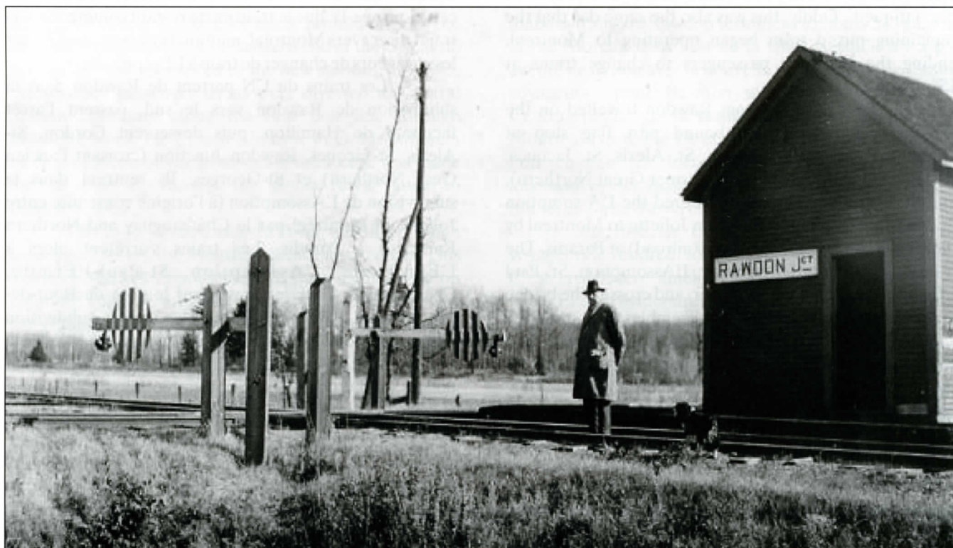
A rare photo of Rawdon Junction, probably taken around 1930. The photographer is facing northwest. The unusual gates are protecting the CNR St. Jerome line by blocking the Rawdon line. Glenn Cartwright collection.
