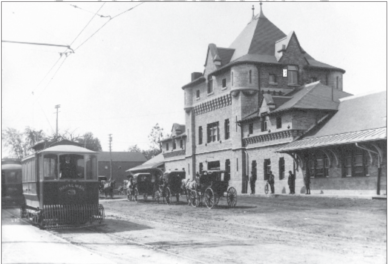
Ottawa Electric Railway Royal Mail car #3 was the third of the horse cars from the Ottawa City Passenger Railway converted to electric mail cars. It stands outside the handsome gothic style CPR Broad Street Station awaiting the arrival of mail from incoming trains. Library and Archives Canada, C 8676.
