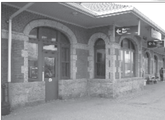
Note the stone and brick detail surrounding the window and door casements of VIA's Cobourg station, a tribute to the masons of a century ago. The telegrapher's bay was part of the original ticket office, but today this area is part of the general waiting room. Ted Rafuse.
