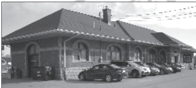
A view snapped from the southwest looking towards the northeast. The first two windows on the south side were part of the original baggage room and remain so. The first window beneath the roof jut was part of the original express room and is now a part of the ticket office. The window adjacent to the vestibule was part of the original general waiting room but now is part of the women's washroom. Ted Rafuse.
