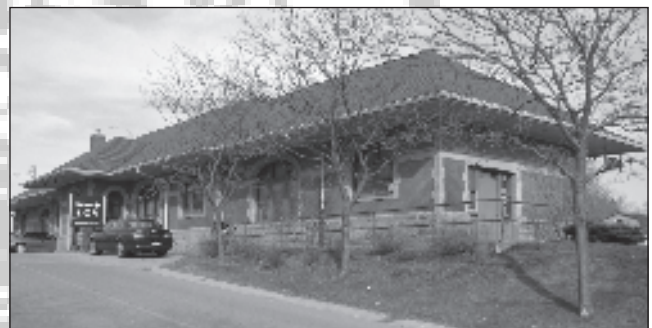
This image looks from the southeast to the northwest. The large window once illuminated the original restaurant but today admits light to unused space. The small window on the end was part of the original kitchen. The smaller window to the left of the large one was once part of the women's washroom in the original women's waiting room section. Surrounded by a windowed casement the door on the east end led to the original kitchen area. Ted Rafuse.
