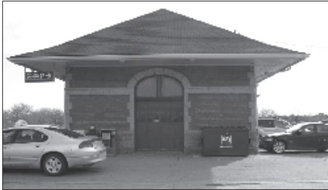
The west façade illustrating the entrance to the baggage room. Ted Rafuse.
