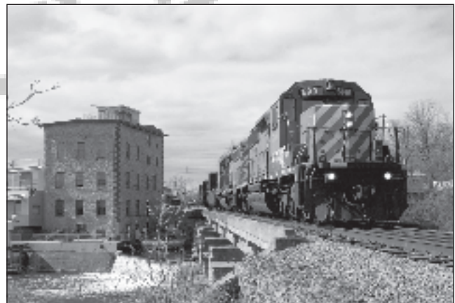
CPR rail lifting train crossing the Mississippi River at Almonte, Ontario on April 18, 2012. Raymond Farand.
