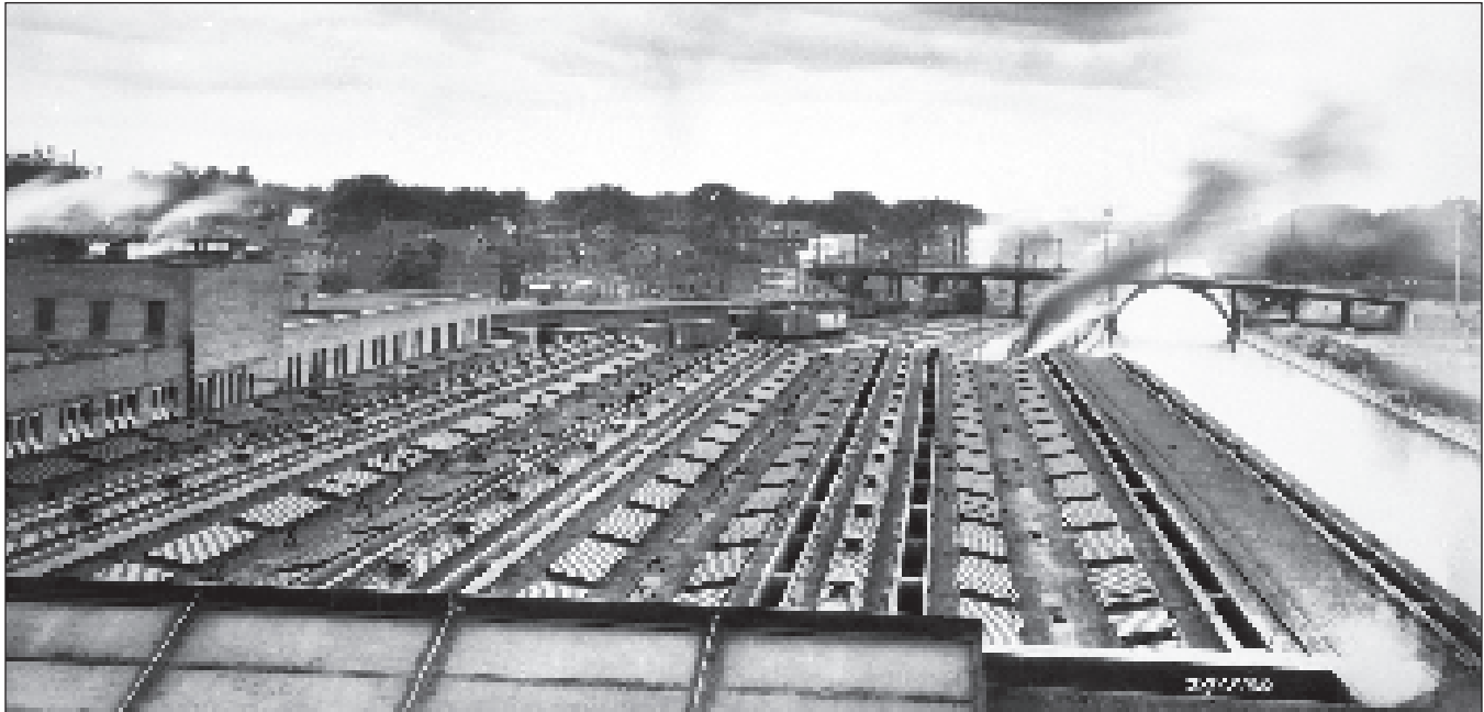
Overview of the train-shed roof of the Ottawa Central Station in 1928. Canada Science and Technology Museum, CN Collection 005681.
