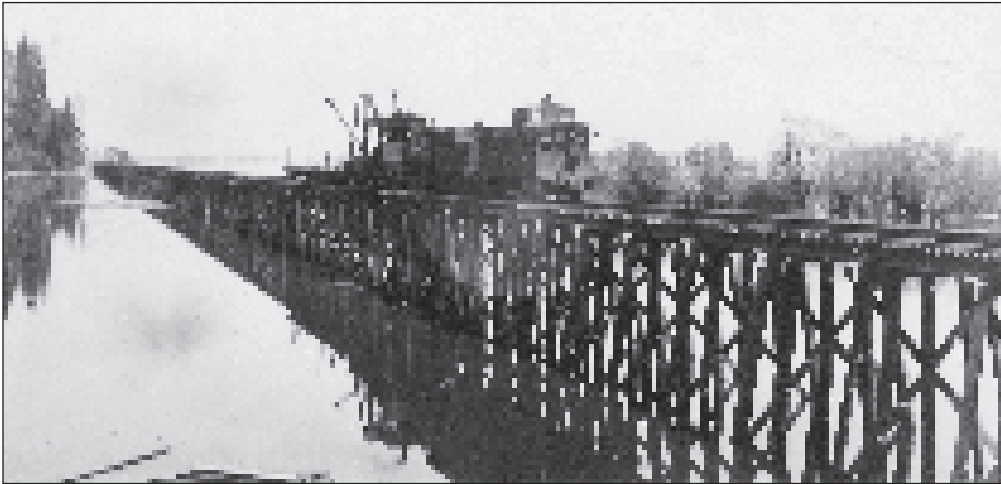
This photo shows a Great Northern work train on the long wooden trestle crossing the outer edge of Sumas Lake at what appears to be where the Sumas River flows now. The lake was drained in 1924. Some remnants of this trestle remain. The Reach Gallery Museum Abbotsford, P3827.
