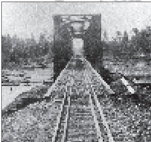
The new Howe wooden truss bridge over the Similkameen River near Keremeos circa 1906. Okanagan Archive Trust Society, GNR 102, www.oldphotos.ca
