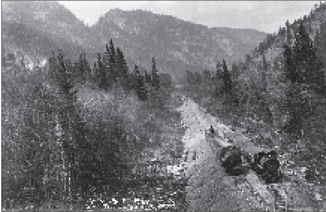
Construction of the Coalmont siding near Otter Lake circa 1910. Okanagan Archive Trust Society, GNR 016, www.oldphotos.ca
