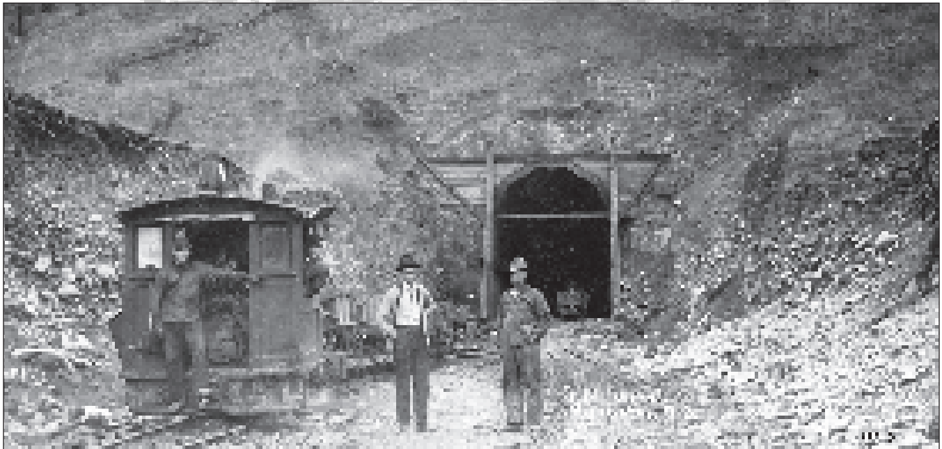
Contractors with their narrow gauge railway equipment digging the Great Northern tunnel west of Princeton, British Columbia circa 1908. Okanagan Archive Trust Society, GNR 002, www.oldphotos.ca
