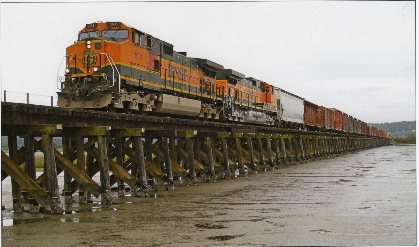
Bridge 70 on the BNSF Railway's New Westminster Subdivision feels the weight of GE C44-9's 1001 and 1116 handling the Pasco-New Westminster mixed freight on September 2, 2007. Bridge 70 is 2700 feet long and is ten miles north of the U.S. - Canada border. Ian Smith.
