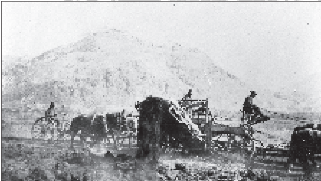
A horse-powered grader at work clearing a Great Northern right-of-way circa 1906. Okanagan Archive Trust Society, GNR 094, www.oldphotos.ca
