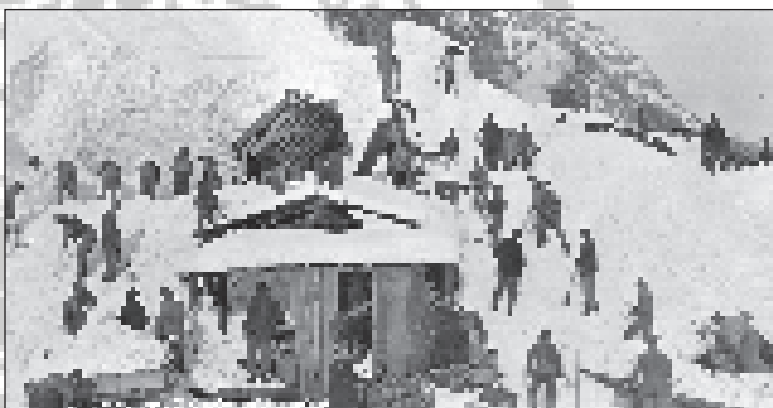
Railway workers digging out from a snowslide in the Coquihalla circa 1915. Kettle River Museum Archives, Midway, British Columbia.
