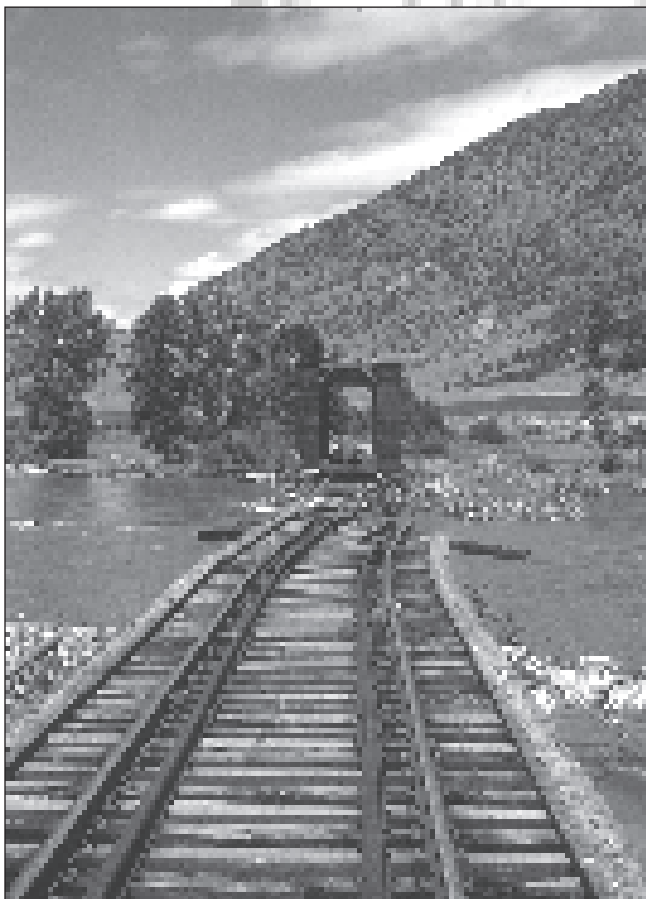
In the spring of 1972, the Similkameen River washed out Bridge 7 which was located just south of Similkameen station. By this time, the only shippers on this segment of Hill's 'Third Main Line' were fruit growers near Keremeos, B.C. Several BN reefers were stranded because of the flooding and were eventually trucked out by 1974 as the GN abandoned the line between Oroville, Washington and Keremeos, British Columbia. The distinctive wooden Howe truss design is evident in these photos from 1972. Philip Mason.
