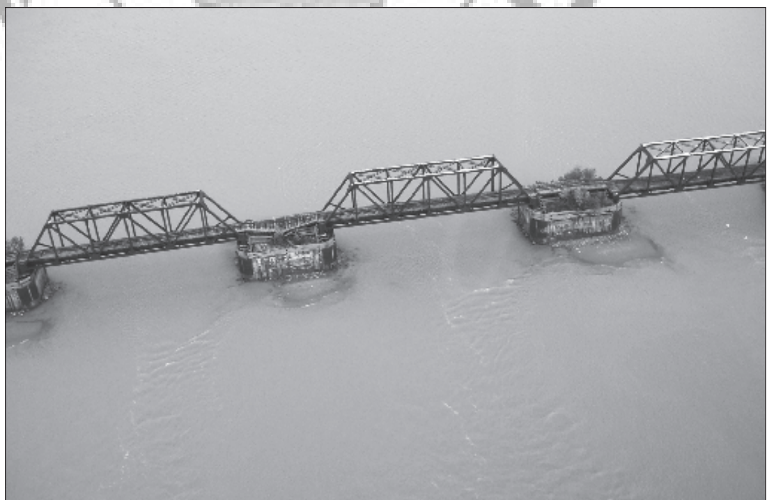
Abandoned rail bridge at Port Nelson showing the ravages of time; sagging rails between spans, July 2010. Thomas Woodcock.
