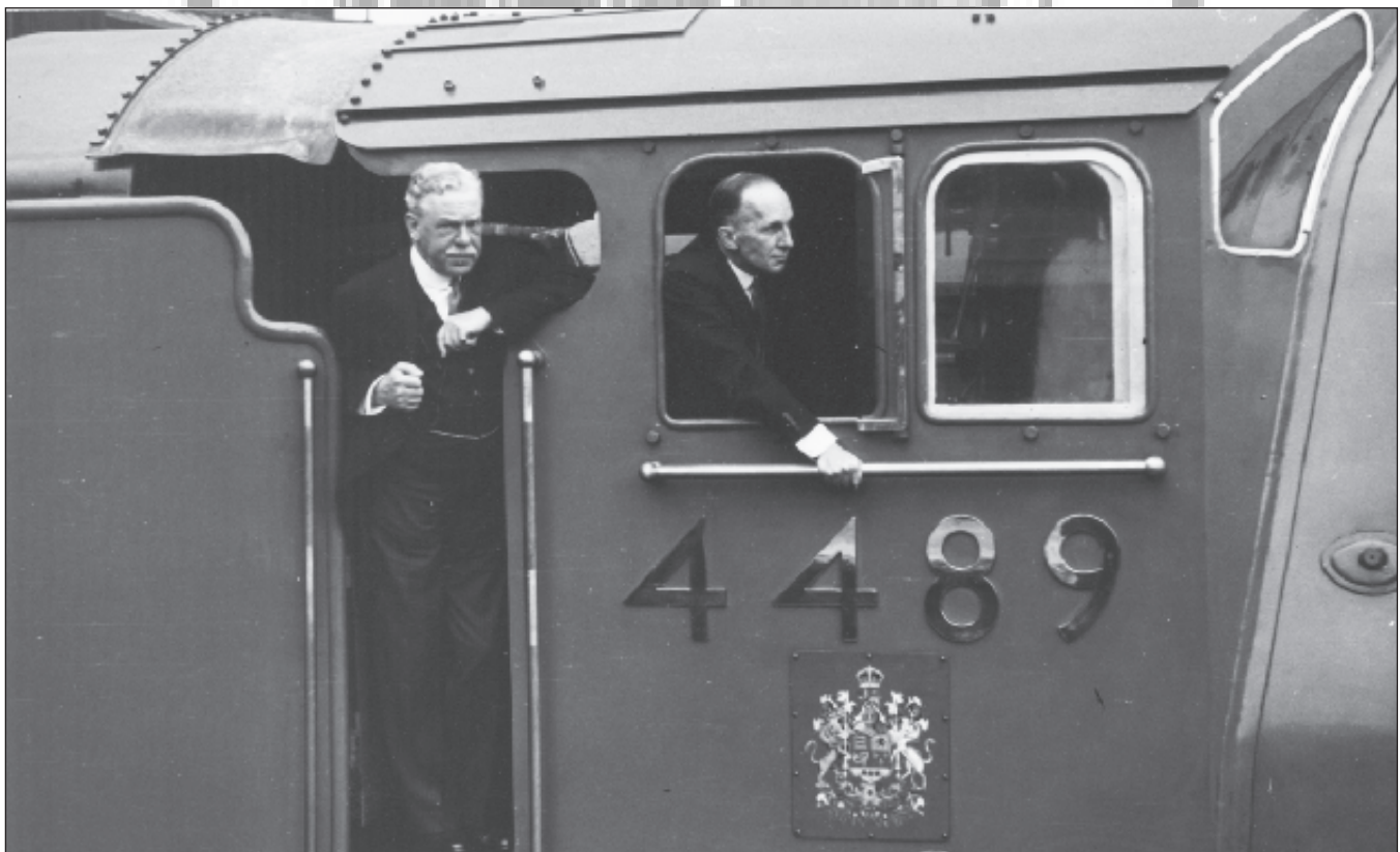
Commissioning in 1937 National Railway Museum / science and society picture library / La mise en service en 1937
