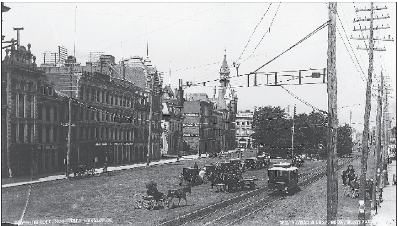
A horsecar heads west on King Street near James St. circa 1890. The electrical bracket and apparatus on the pole is to support the carbon-arc street lamp. The newer horsecars would soon be converted to electric propulsion instilling fear in some of the riders! William Notman and Son, the McCord Museum View-2304
