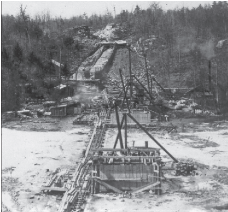
This construction image captures the cribbing around the caissons for the middle and west bridge piers. The photo was probably taken in winter 1912-13. Note the small rail system on the temporary bridge over the frozen Mud Lake, the plant boiler to the right and various small buildings, the bunkhouses for the workers and several stiff-leg derricks for hoisting material into place. To the left of the pier is a man walking thereby providing a perspective suggesting the size of the project being undertaken. Image courtesy Jessie Donnelly
