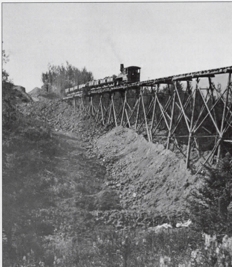
Filling in one of the many temporary wooden trestles on the GTP. Glenbow Archives NA-3658-33
