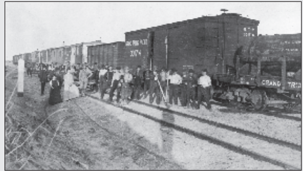
Once the tracks were laid and ballasting done, the fencing crew secured the right-of way. Glenbow Archives NA-3304-4
