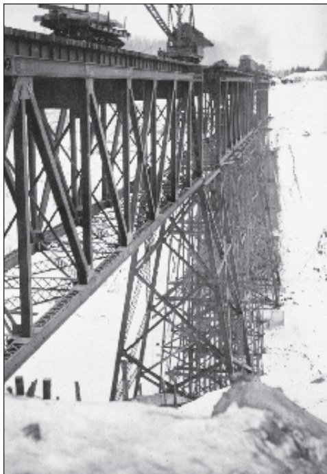
Grand Trunk Pacific Railway steel bridge over the Pembina River in Alberta. Glenbow Archives NA-945-25
