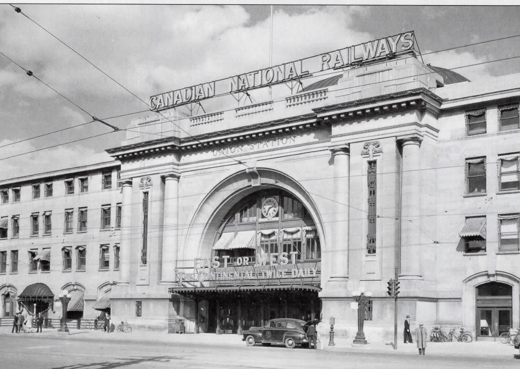
Union Station was designed by Warren and Wetmore, the architects responsible for Grand Central Terminal in New York City. Designed in the Beaux-Arts style and constructed from local Tyndall limestone, Union Station was one of Western Canada's largest railway stations. Canada Science and Technology Museum
