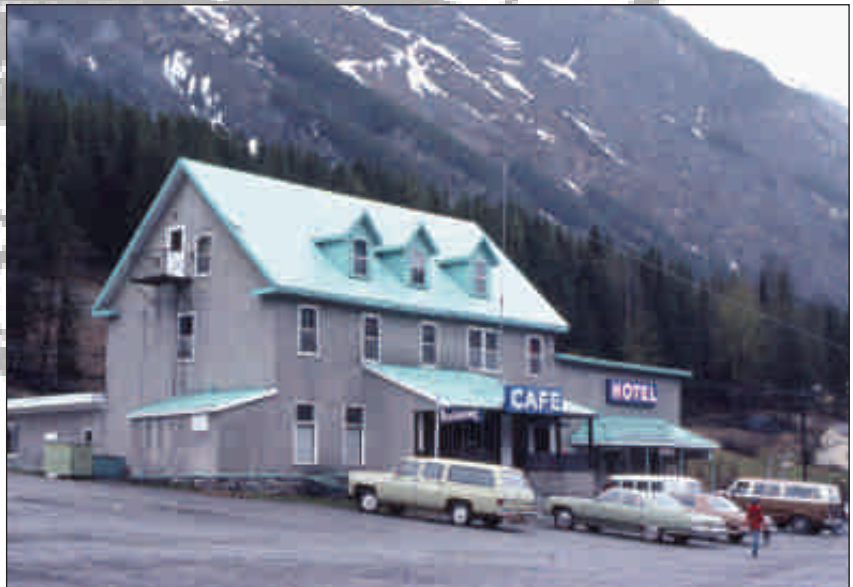
In May 1976 the Monarch Hotel was still serving railroaders and others. The roof-top sign had disappeared but true life railroad stories could still be heard in the beer parlour of the Monarch! Joanne MacPherson, Smaill collection
