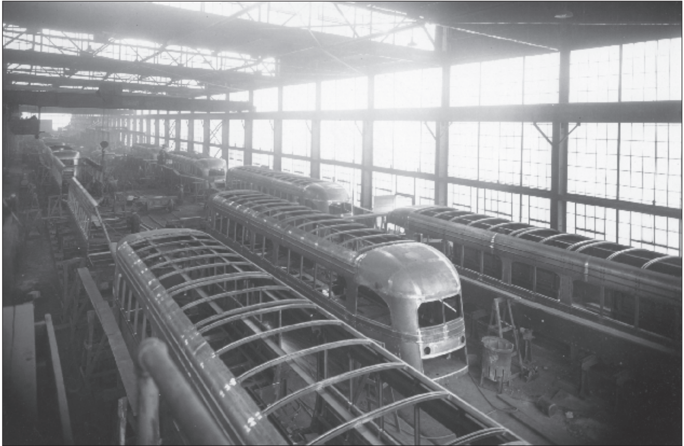
The fabrication of PCC bodies is in full swing at the St. Louis Car Company's erecting shop circa 1938. Washington University in St. Louis, Special Collections - St. Louis Car Co.
