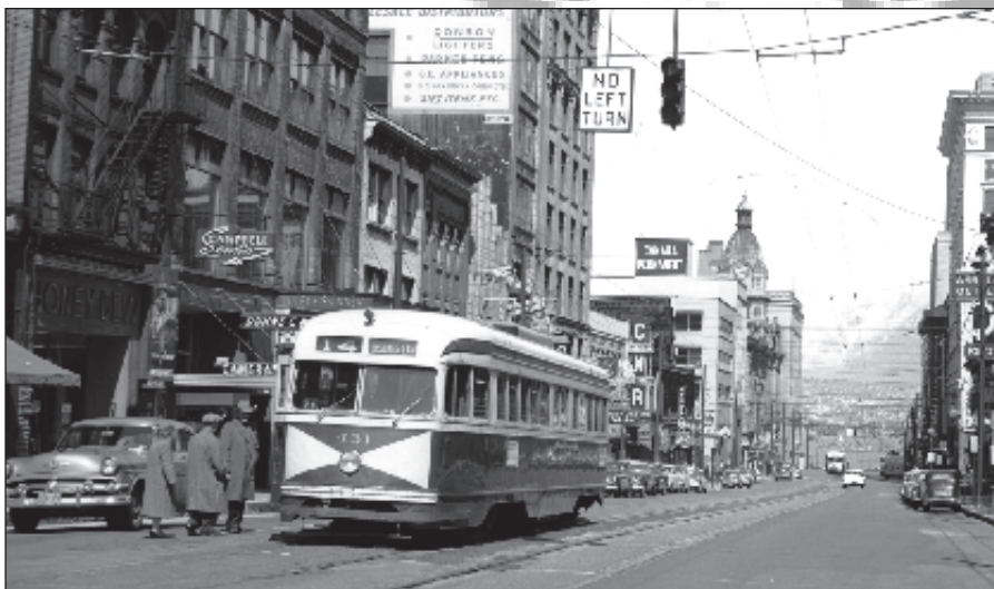
BCER 431 is southbound on Granville Street between Pender and Dunsmuir Streets on April 18, 1955. Stan Styles, GTC Collectibles BCE-431-1
