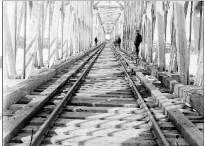
Two views of Mackenzie's impressive wooden bridge over the South Saskatchewan River at Saskatoon on the Qu'Appelle, Long Lake & Saskatchewan Railway circa 1890. Most of the bridge was destroyed by an ice-jam in 1904. Saskatoon Public Library LH-3092 and LH-24
