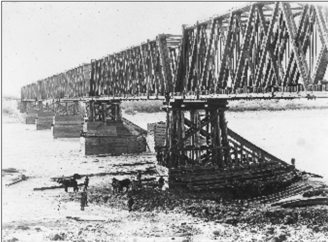
Two views of Mackenzie's impressive wooden bridge over the South Saskatchewan River at Saskatoon on the Qu'Appelle, Long Lake & Saskatchewan Railway circa 1890. Most of the bridge was destroyed by an ice-jam in 1904. Saskatoon Public Library LH-3092 and LH-24
