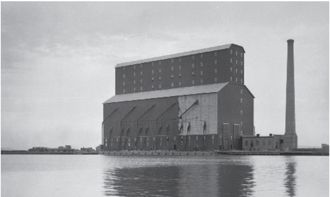
To reach deep water, CNoR's elevator was built several hundred feet out from the lakeshore and was accessed over a long trestle. Library Archives Canada PA-026106
