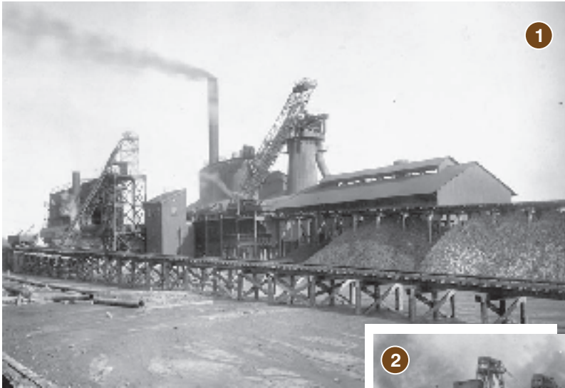
Atikokan Iron Company's smelter at Port Arthur functioned intermittently from 1907 to 1911. Library and Archives Canada PA-021147
