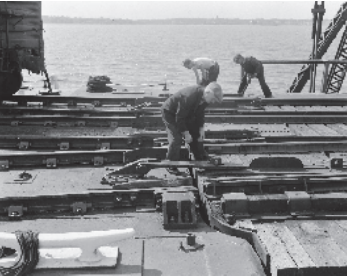
Workers busy docking the Prescottont at Prescott, Ontario in August, 1948. This is a good view of the rail arrangement on the dock and ferry. Roger Robinson, CRHA Archives, Fonds Canadian Pacific
