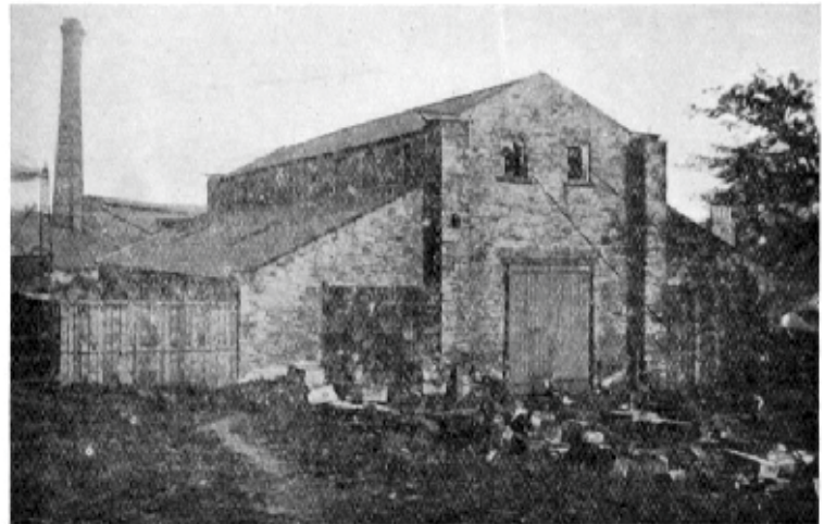
Timothy Hackworth's Shildon erecting shop. (Hackworth website) L'atelier de montage de Timothy Hackworth à Shildon. (Site Internet Hackworth)
