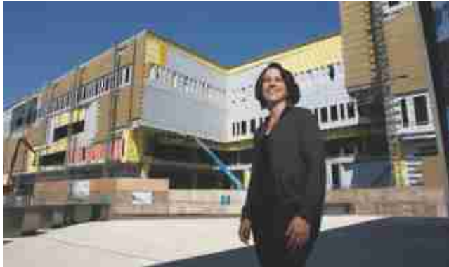
Ingenium president Christina Tessier in front of the new storage facility under construction. (Blair Gable)
