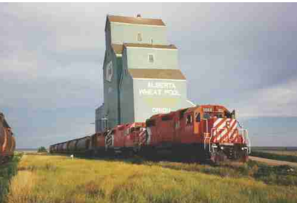
View of the last elevator of the former row at Orion, Alberta in September 1998. A few weeks after the last westbound grain left Orion, the elevator was closed. Within a year the elevator would be demolished and the track from Orion to Etzikom would be removed by CPR. Nick Korchinski collection, Great Canadian Plains Railway Society / Galt Historic Railway Park archives
