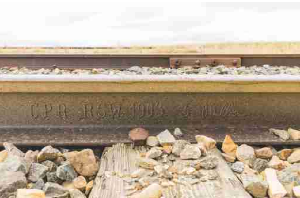
View of 1903 German steel (Rheinische Stahlwerke AG) on the elevator track at Skiff, Alberta in April 2014. Jason Sailer
