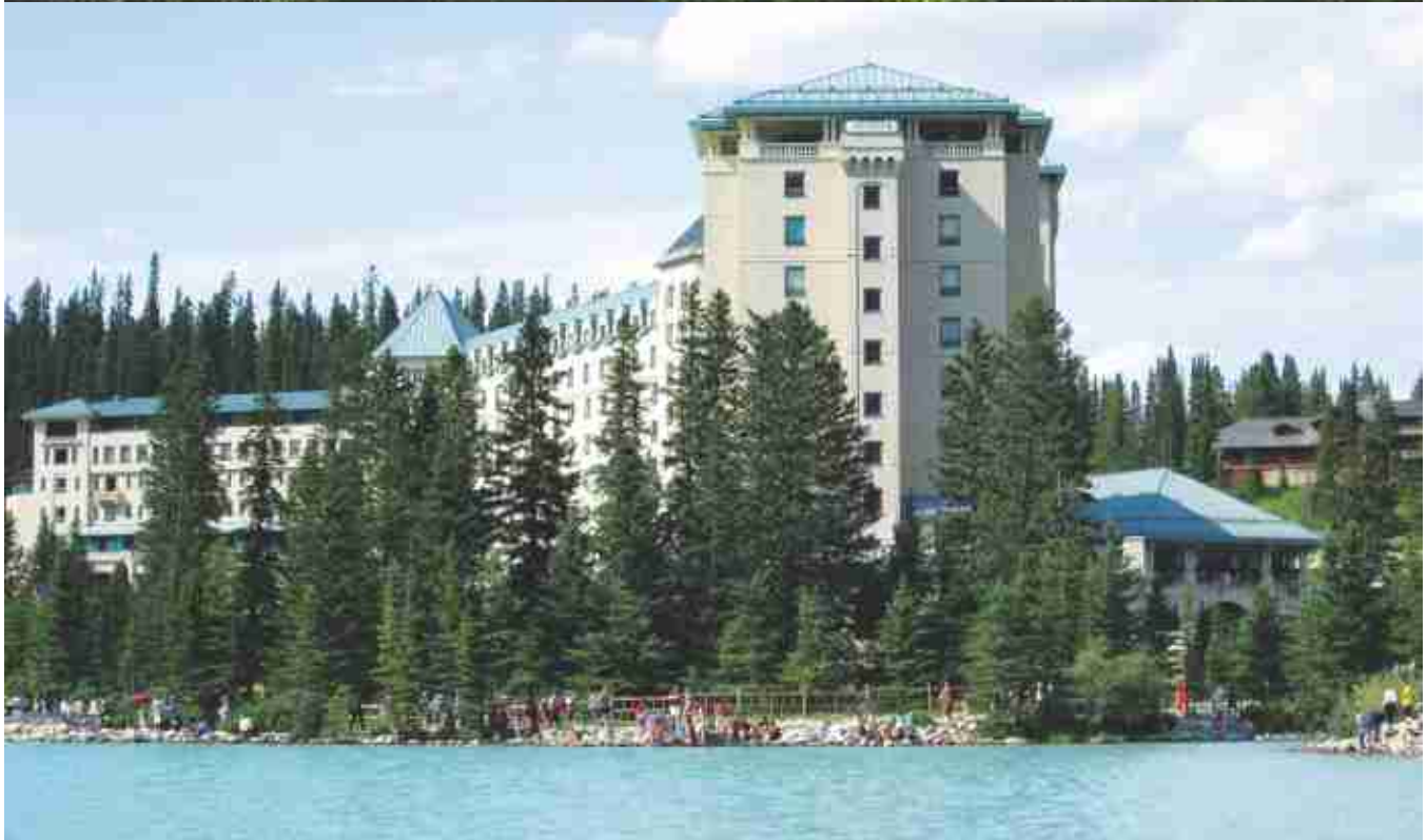
Two of the crown jewels in Canada's former railway hotel chain are the Banff Springs Hotel (1886) and Chateau Lake Louise (1890), both survive as Fairmont properties. Garth Stevenson
