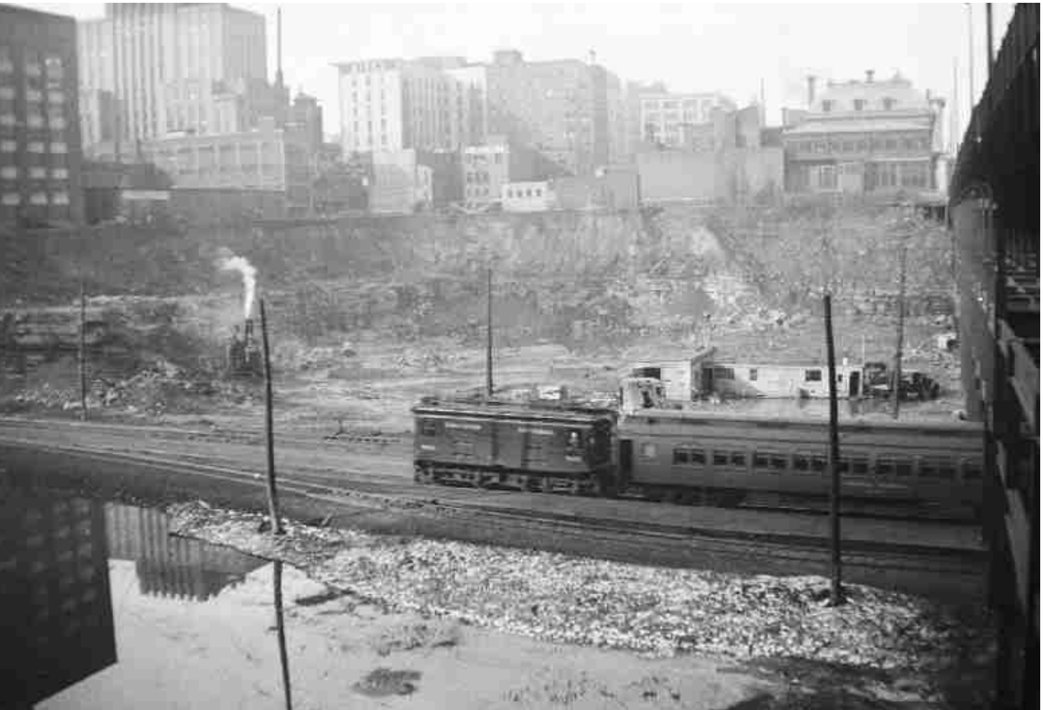
A commuter train hauled by CN 9103 leaves Tunnel Terminal towards the Mount Royal Tunnel on March 18, 1947. Excavation has already begun on the lead tracks from the tunnel to Central Station. Place Ville Marie covers this view today. CRHA / Exporail Archives, Fonds Ronald S. Ritchie - Ernest L. Modler Collection 1453
