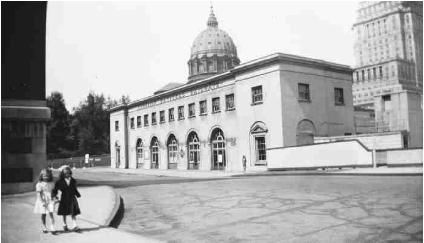
View of Canadian Northern Railway's Tunnel Terminal from Lagauchetière Street. Mary Queen of the World Basilica and the Sun Life building grace the background. CRHA/ Exporail Archives, Fonds Ronald S. Ritchie - Ernest L. Modler Collection 3821
