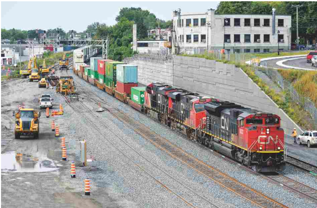
Nearing completion. The massive track diversion of the CN Montreal Subdivision as a result of the Turcot Expressway reconstruction project in Montreal is just about complete in this August 27, 2018 photo. CN 8833 East has train 120 bound for Halifax operating on the new right of way alignment at Turcot Ouest. Ken Goslett
