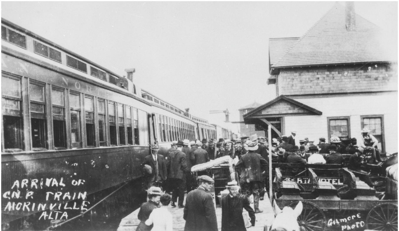
After reaching Edmonton late in 1905, the CNoR started construction of a branch northwards to the Athabasca River. Morinville, 26 miles from Edmonton, was reached in 1906. Alberta Archives, A15474
